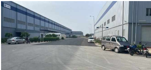
Indo Space Industrial & Logistics Park. Faizabad, Tehsil-Badli – Jahajjar (Sr No 37)
