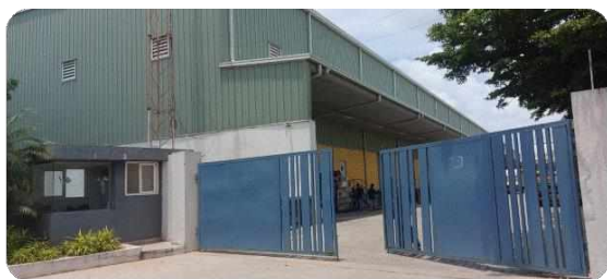
Survey-643/B, Devaramzal Village, Shamirpet, Malkajgiri Dist – Hyderabad (Sr 7)
