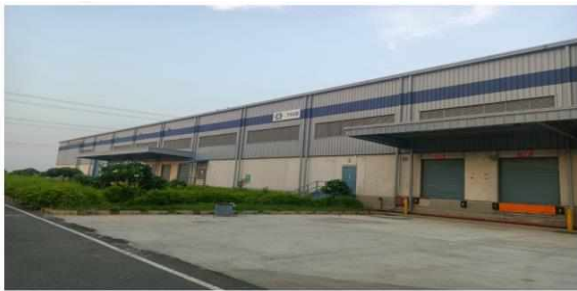
Unit no.A Building No. B750 (Hcy Industrial Park Pvt ltd, Indo space Logistics Park ,Luhari, Jhaajjar (Sr No 29)
