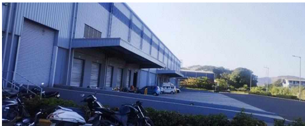
Building No B200, Shed 200, Indran Logi Indospace Industrial & Logistics, Ajivali, Khalapur Raigad - Khopoli (Sr No 21)
