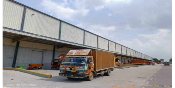
Embassy Industrial Park, 122506 Farukhnagar – Haryana (Sr No 28)
