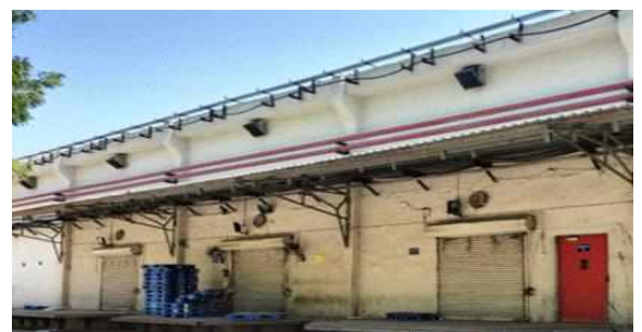
Gate No 5,GIDC Naroda - Ahmedabad (Sr 17)
