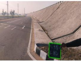
Fig 4.179: RCC Toe Drain at Ch 47+140 LHS
