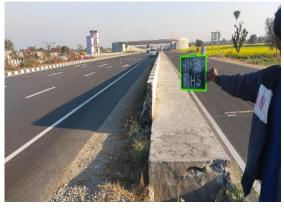
Fig 4.174: RCC Toe Drain at Ch 41+300 RHS
