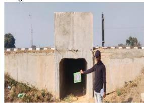
Fig 4.362: Box Culvert at Ch 43+480 LHS
