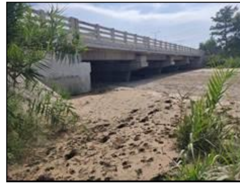
Minor Bridge at km. 68+519 (New Structure View)
