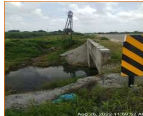
Box culvert at km. 105.290 - RHS (New Construction)
