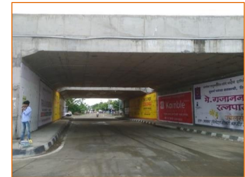
Light Vehicular Underpass at km. 298.613
