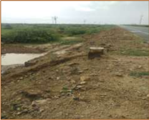
HPC at km. 487+054 (LHS)
