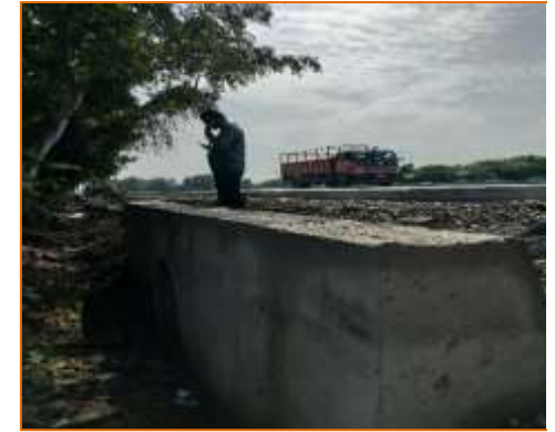
HPC at km. 32+520 (LHS)
