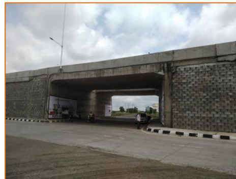
Vehicular Underpass at km. 292.758
