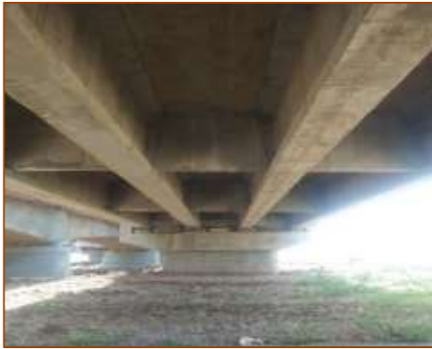
Bottom of MJB - New at km. 433+276 (LHS)
