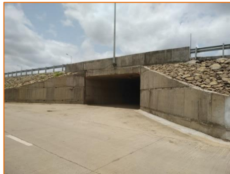
Pedestrian Underpass at km. 284.500
