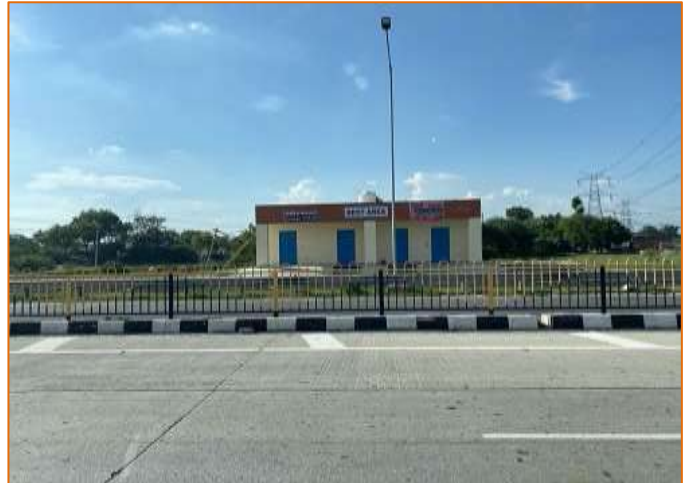
Rest Area at km. 767+500
