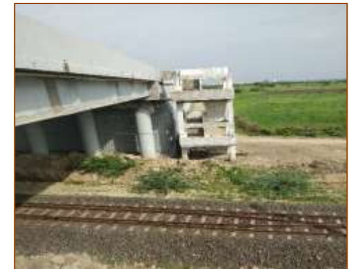
Side View of ROB at km. 393.642 (LHS)
