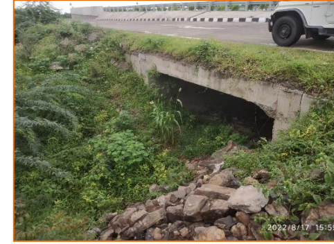
Box Culvert at km. 311.734
