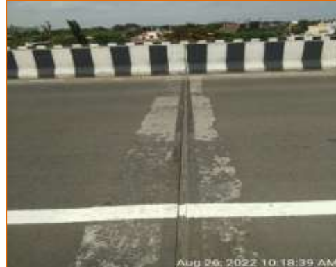
Filled expansion joint of Flyover at km. 130.650 (RHS)
