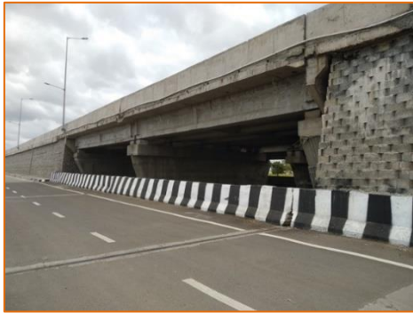
New Minor Bridge at km. 288.035
