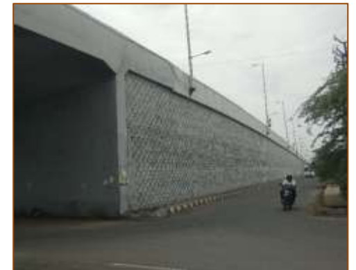
VUP at km. 400+681 (LHS) at A1 side
