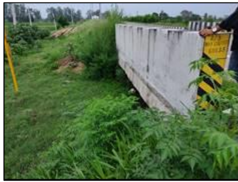
Box Culvert at km. 1+457
