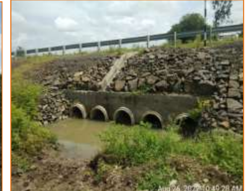
Pipe Culvert at km. 124.106-LHS (Widening)
