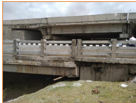
New Minor Bridge at km. 292.148
