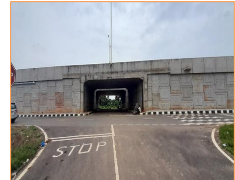
View of LVUP at km 61+932
