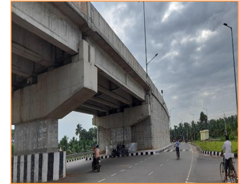
View of UDFO at km. 48+830
