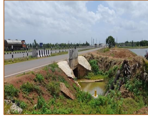
Box Culvert at km. 35+736
