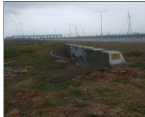
HPC at km. 409+195 (LHS)
