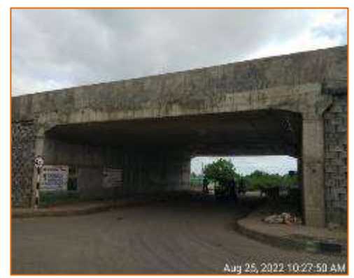
Side View of LVUP at km. 135.100 (RHS)
