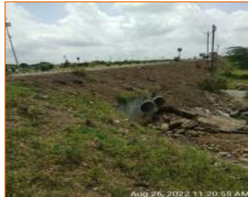
Pipe Culvert at km. 117.423 - LHS (Widening)
