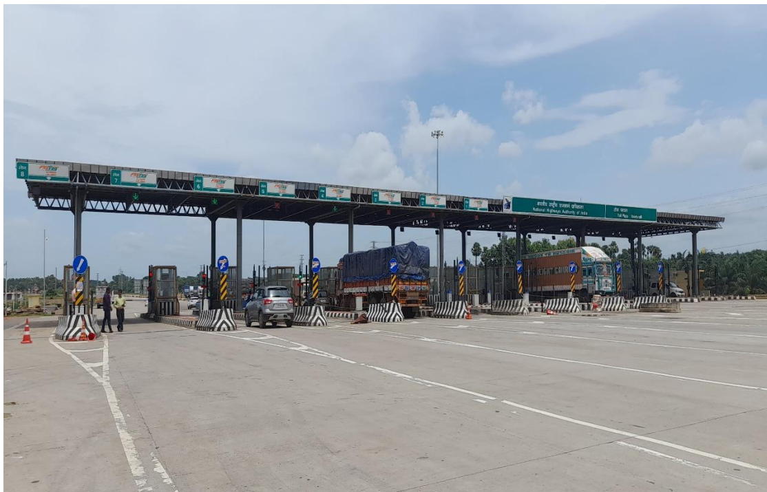
Figure 9-1 View of Toll Plaza (km. 53+700)
