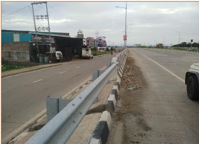
Crash Barrier at km. 285+650
