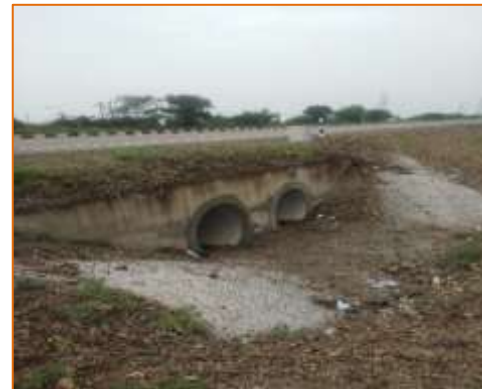
HPC at km. 70+640 (RHS)
