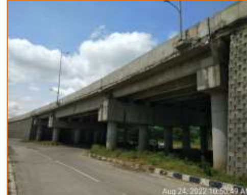
Side View of Flyover at km. 99.900 (RHS)
