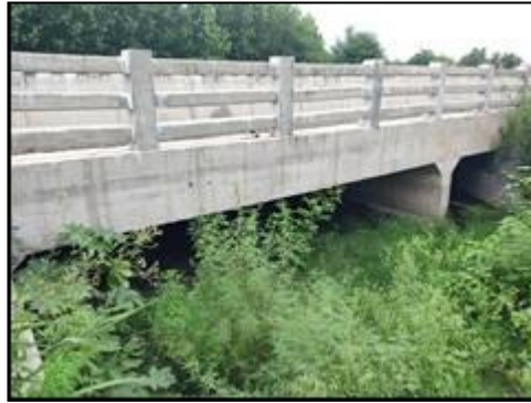
Minor Bridge at km. 74+361 (Structure View)
