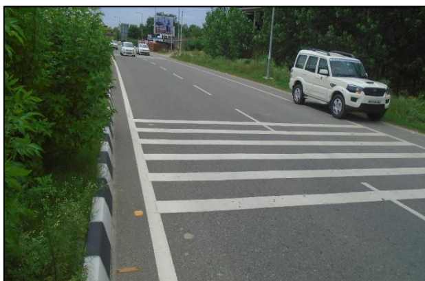
Road Marking at km. 70+000 (RHS)
