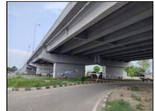
Flyover at km. 9+335
