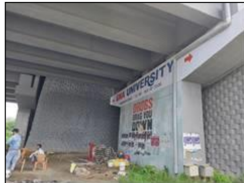
Flyover at km. 4+225
