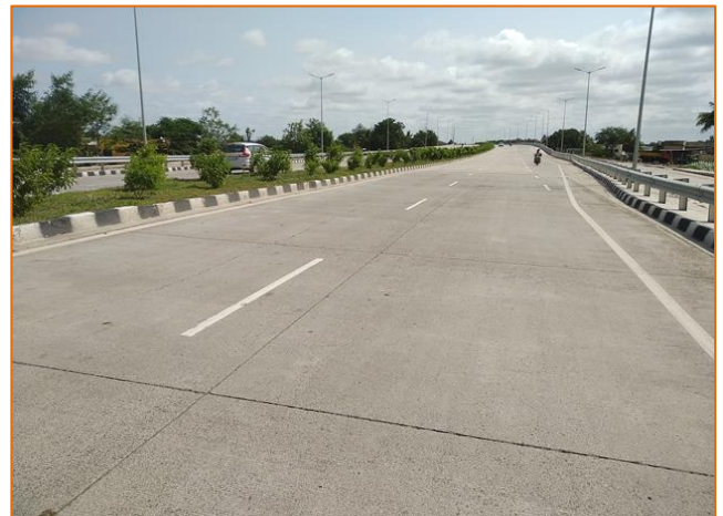
Start of Project Road at km. 276.000
