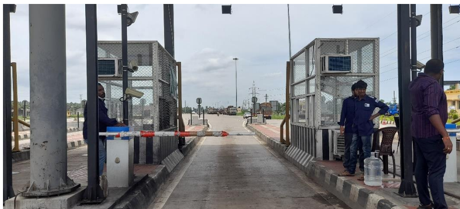
Figure 9-6 Automatic Lane Barrier
