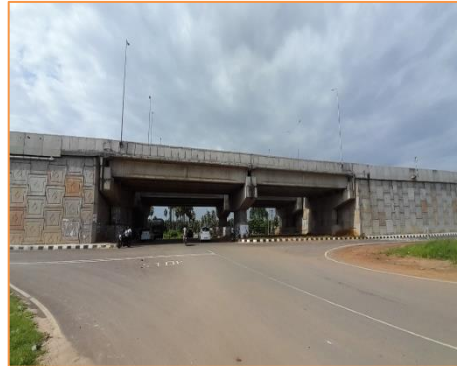
View of Flyover at km. 45+645
