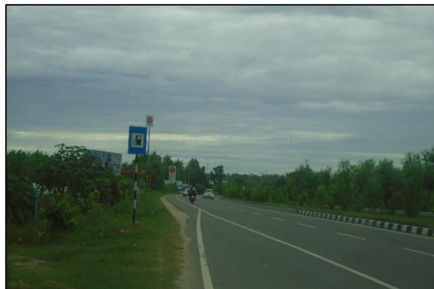
Traffic Sign Board at km. 72+000
