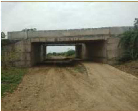
LVUP at km. 422+750 (RHS) - Under COS
