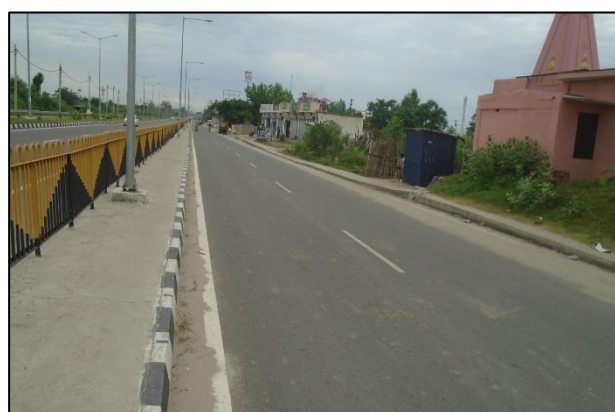
Service Road at km. 77+600 (LHS)
