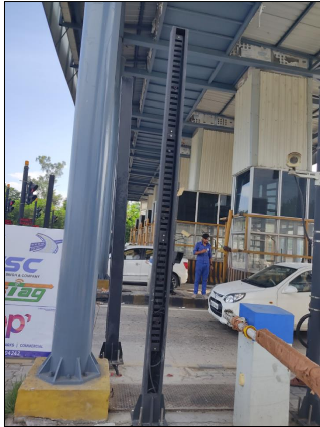
Figure 9-5 Height sensors
