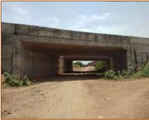
LVUP at km. 381+600 (RHS) - Under COS
