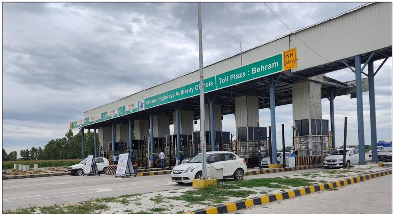
Figure 9-1 View of Behram Toll Plaza (km. 15+300)
