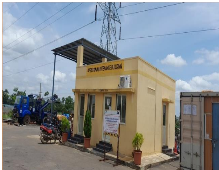
Figure 3-20 Operation and maintenance building at Toll Plaza
