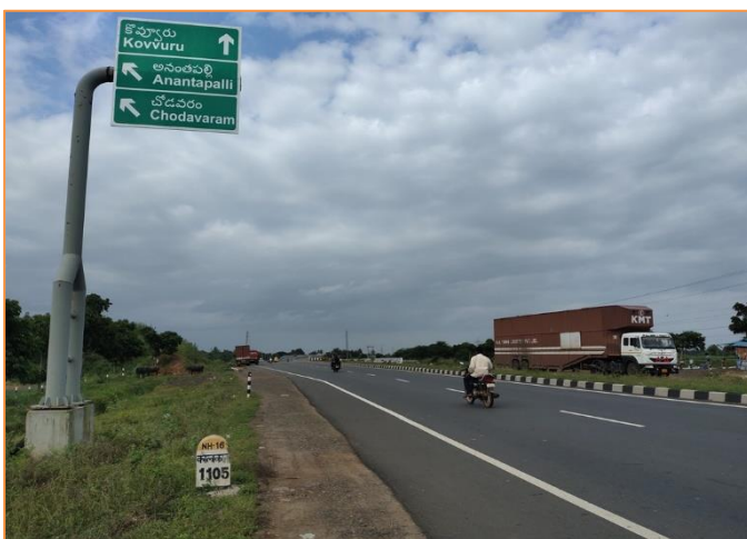
Cantilever Sign at km. 67+000
