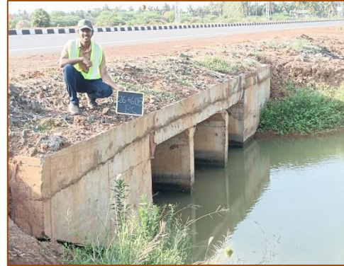
Box Culvert at km. 26+605
