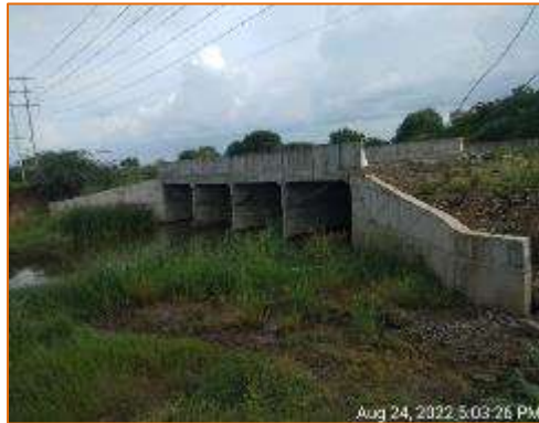
Side View of MNB at km. 99.586 (RHS)
