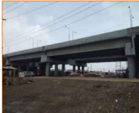
Side View of VUP at km. 12+420 (LHS)
