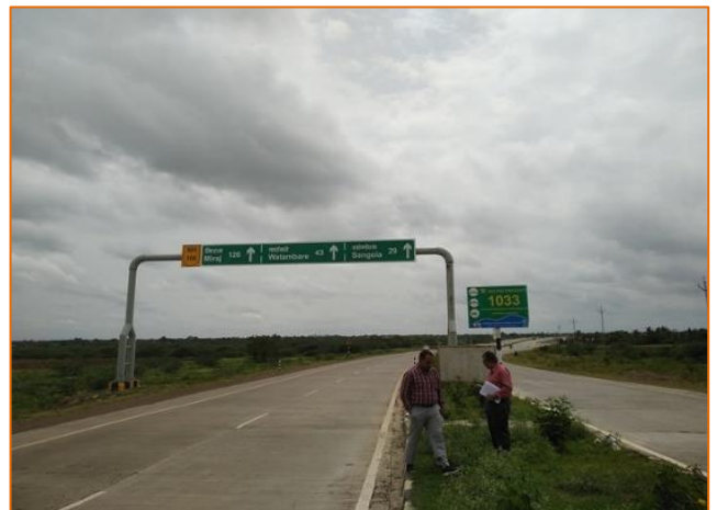
End of Project Road km. 321.600
