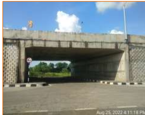
Side view of LVUP at km. 111.260 (LHS)
