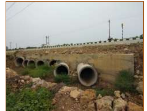
HPC at km. 456+200 (RHS)
