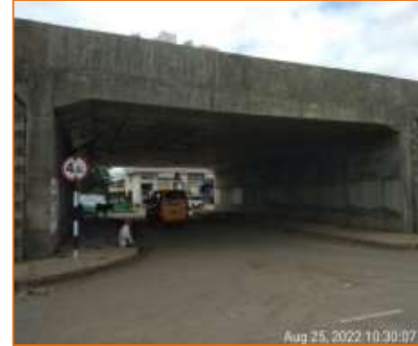
Side View of LVUP at km. 135.100 (LHS)
