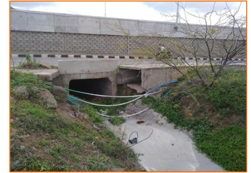
Box Culvert at km. 285+300
