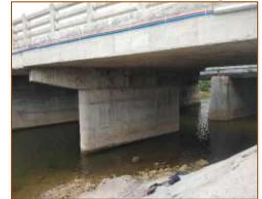
Bottom of Minor Bridge at km. 455+195 (RHS)
