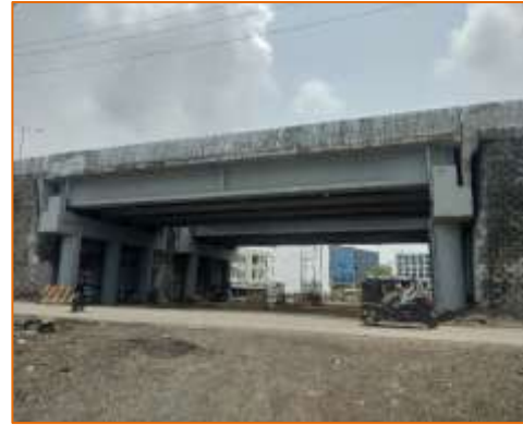
Side View of VUP at km. 58+570 (LHS)
