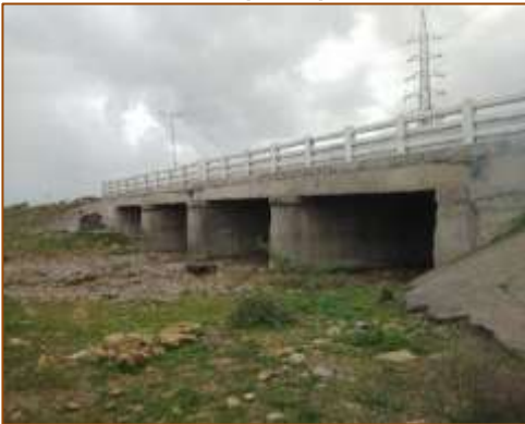
Side View of Minor Bridge at km. 462+447 (LHS) - Widening
