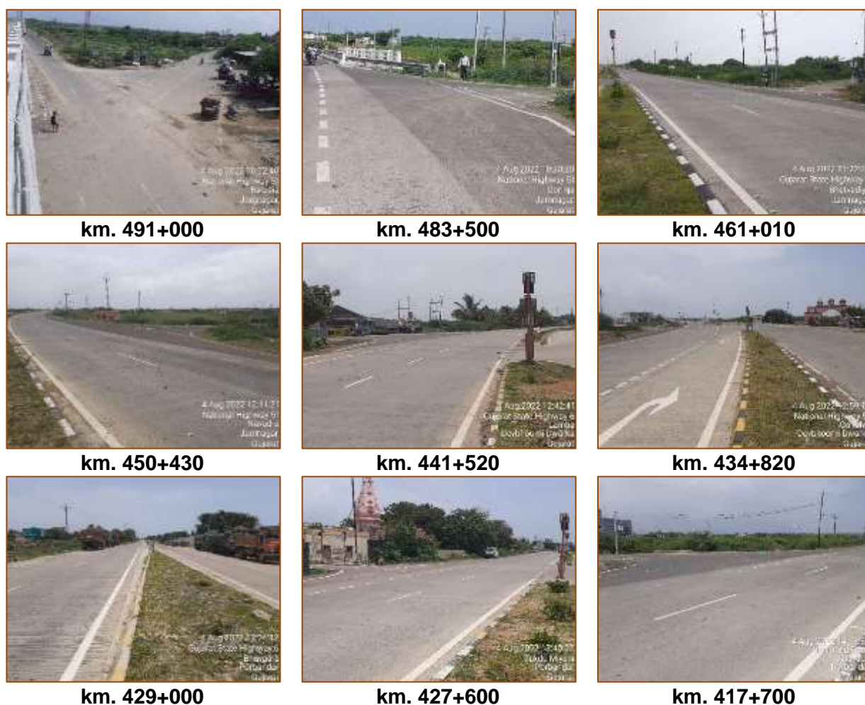
Figure 3-4 Photographs of Minor Intersection
