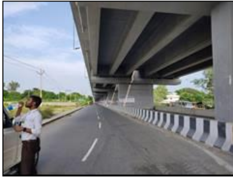
Elevated Structure at km. 25+319
