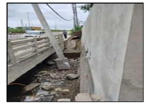
Minor Bridge at km. 80+045 (Structure View)
