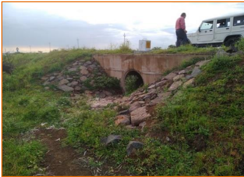
Pipe Culvert at km. 300+020
