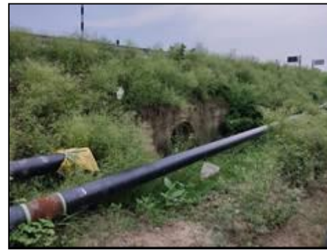
HP Culvert at km. 1+135
