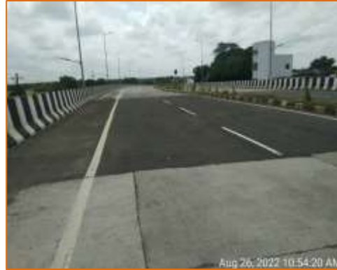
LVUP at km. 121.950 (RHS)
