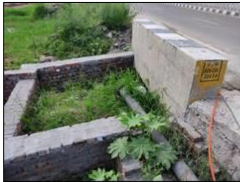
Box Culvert at km. 6+650
