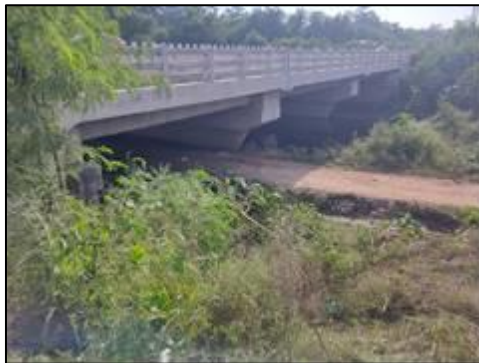
Minor Bridge at km. 71+174 ( Structure View)
