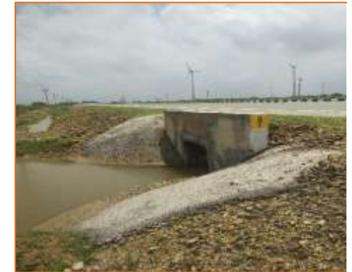
Box culvert at km. 7+240 (RHS)
