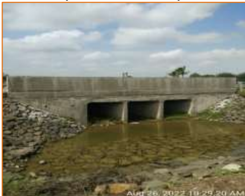
Box culvert at km. 128.229 - RHS (Reconstruction)
