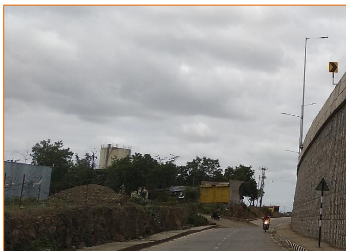
Start point of Sangola Bypass at km. 287+050
