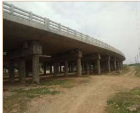
Side View of Major Bridge at km. 422+314 (RHS)
