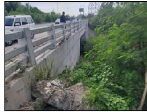
Minor Bridge at km. 69+815 (New Structure View)
