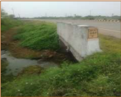
Slab culvert at km. 439+458 (LHS)
