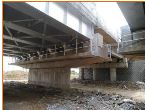
Rail Over Bridge at km. 294.125
