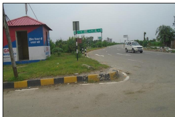
Start of Project Road - Right Carriageway
