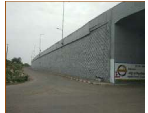
VUP at km. 396+865 (RHS) - A1 side
