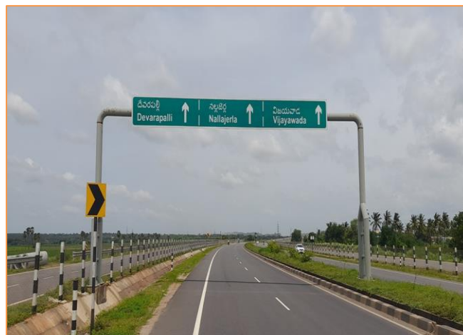
End of Project Road km. 85+204
