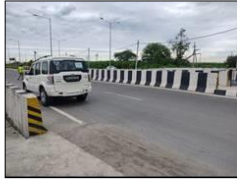
Minor Bridge at km. 77+613 (Top View)
