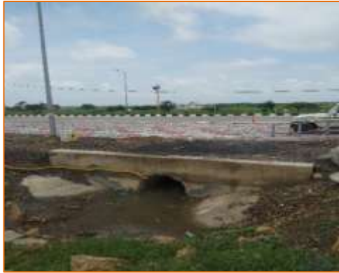
HPC at km. 5+800 (RHS)
