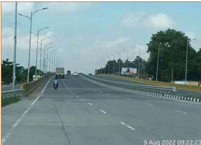
Highway Lighting at km. 773+100
