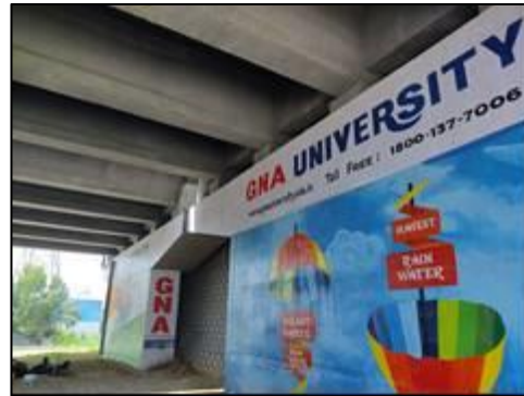
Flyover at km. 39+915
