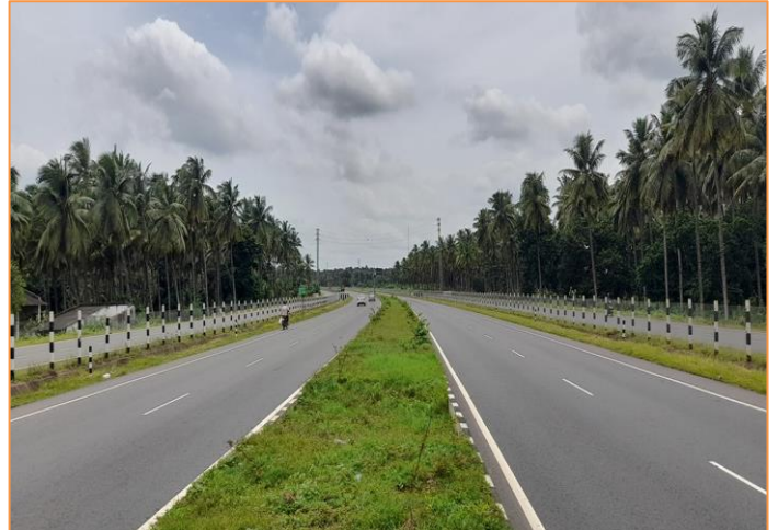
Pavement Condition at km. 46+700
