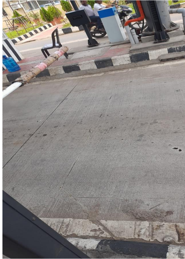
Figure 9-5 Inductive loop
