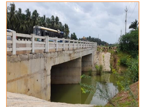
View of Minor Bridge at km. 30+774
