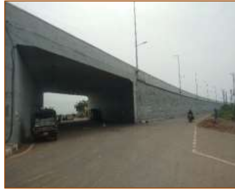
VUP at km. 432+050 (LHS) - (Miyani) under COS - RE Block Wall at A1 side
