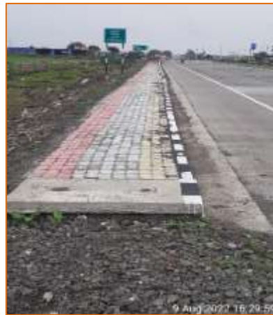
km. 50+000 to km. 49+000 (RHS)
