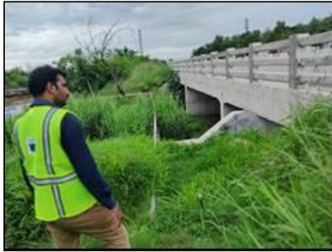
Minor Bridge at km. 74+173 (Structure View)
