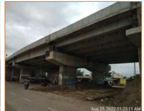
Side View of Flyover at km. 130.650 (RHS)
