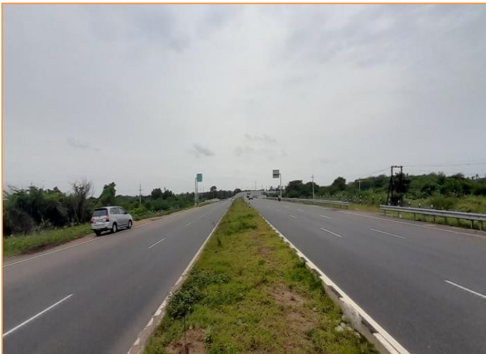
Pavement Condition at km. 55+100
