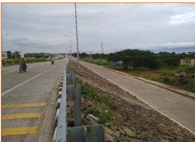
Slope Protection work at km. 284+500.000
