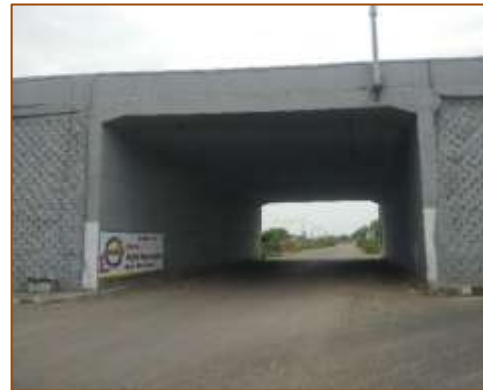
VUP at km. 396+865 (RHS)
