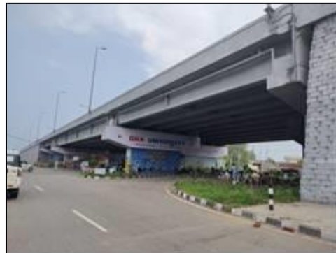
Flyover at km. 4+225
