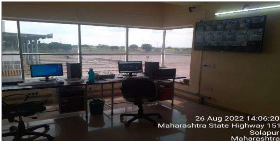
Figure 9-10 Incident Management Workstation at Control room
