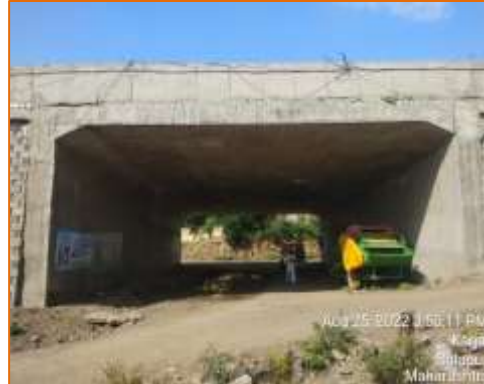
Side view of LVUP at km. 114.080 (LHS)
