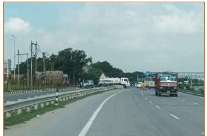
Crash Barrier at km. 782+000
