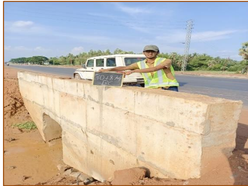
Box Culvert at km. 30+874
