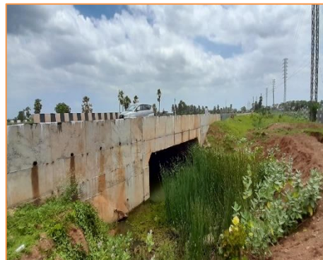
View of Minor Bridge at km. 26+850
