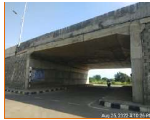
Side view of LVUP at km. 111.260 (RHS)
