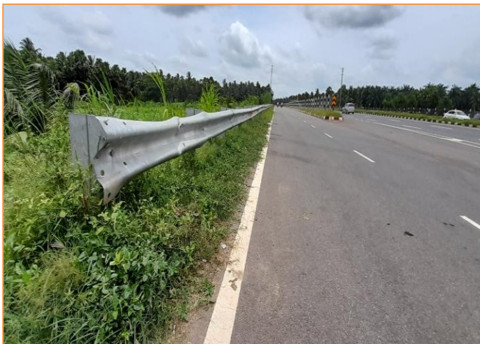
W beam Crash Barrier at km. 52+300
