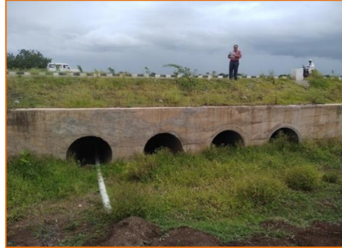
Pipe culvert at km. 317.979
