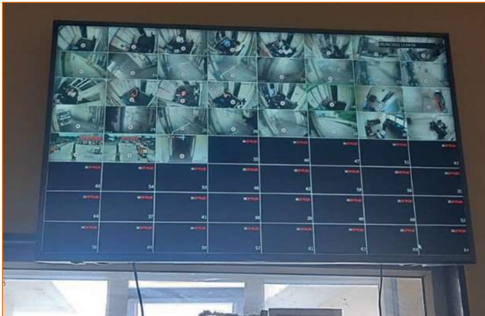
Figure 9-5 55" LED screen for CCTV monitoring
