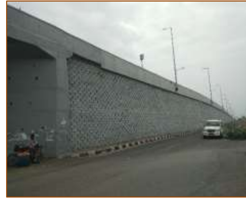
VUP at km. 397+096 (LHS) - Skew - A1 side
