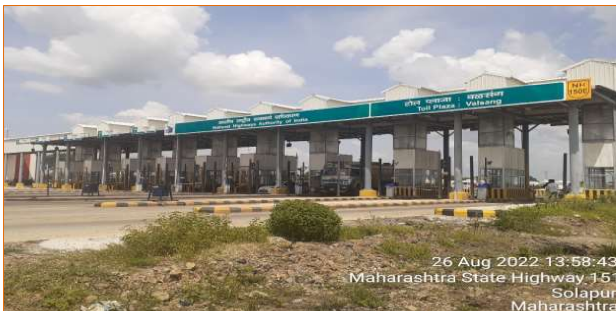
Figure 9-1 View of Valsang Toll Plaza
