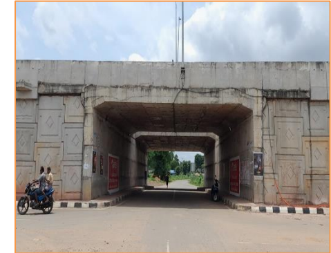
View of LVUP at km 71+140
