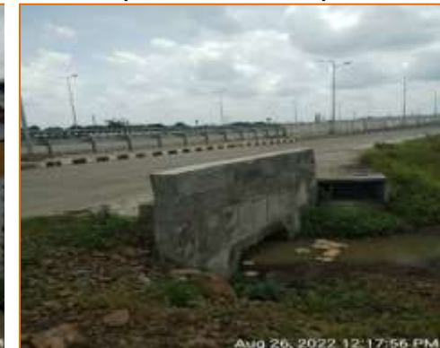
Box culvert at km. 133.524 - LHS (Reconstruction)
