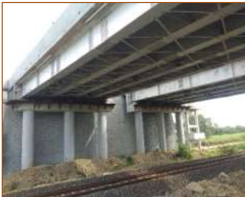
Side View of ROB at km. 393+642 (RHS)
