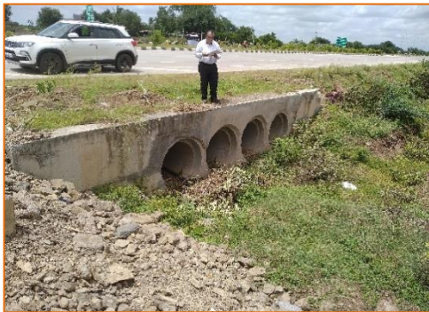
Pipe Culvert at km. 276+190
