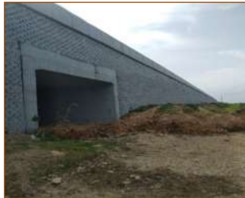
VUP at km. 393+695 (RHS)
