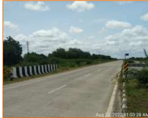
PQC of Minor Bridge at km. 101.260 (RHS)
