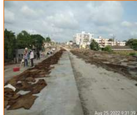
DLC & PQC of Flyover is in progress at km. 136.857 @ Solapur side (BHS)
