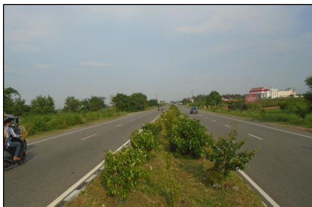
Median Plantation on project highway
