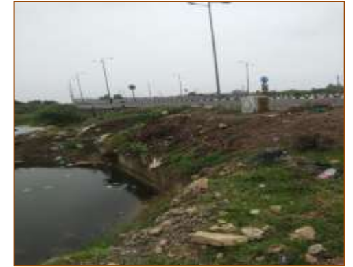
HPC at km. 391+096 (RHS)
