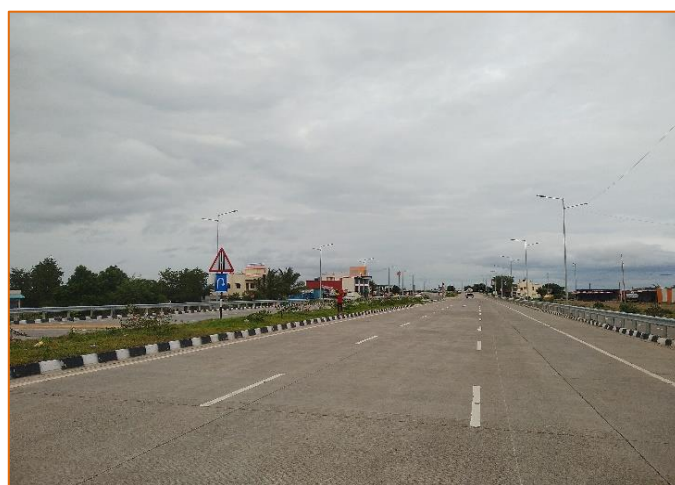
Road Markings at km. 286+600
