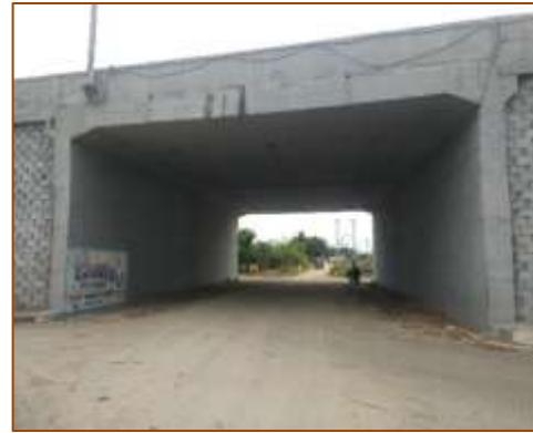
LVUP at km. 422+750 (LHS) - Under COS
