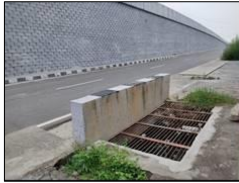
Box Culvert at km. 2+531
