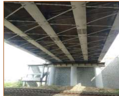
Bottom View of ROB Girder at km. 393+642 (LHS)
