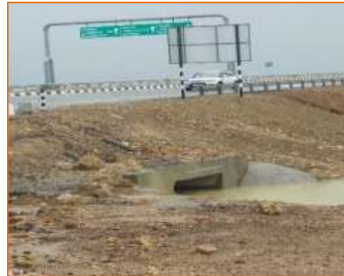
Box culvert at km. 0+060 (RHS)
