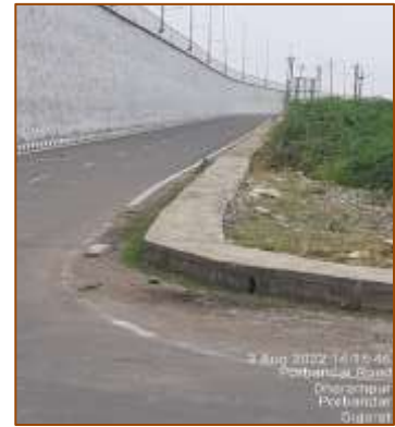
Built-up drain from km. 390+170 to km. 390+953 (LHS)
