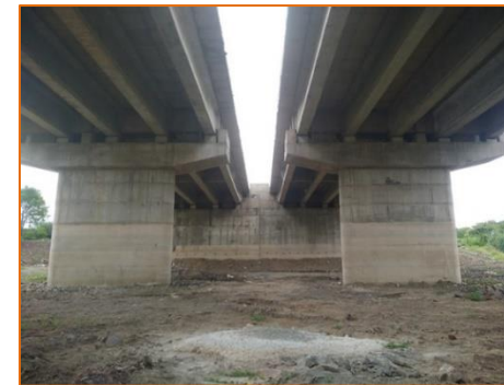
New Major Bridge at km. 298.190
