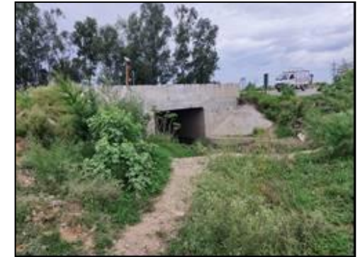
Box Culvert at km. 10+481
