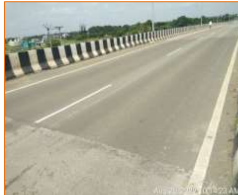
Good BC surface of LVUP at km. 132.025 (LHS)
