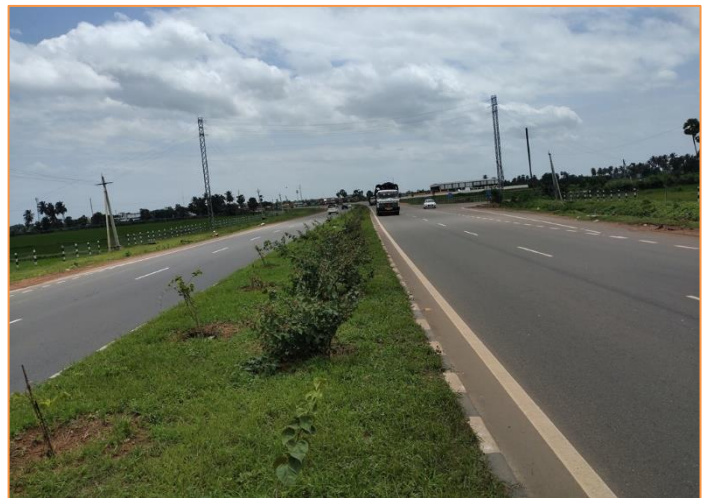
Pavement Condition at km. 57+200
