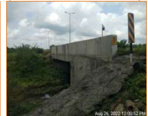
Box culvert at km. 105.290 - LHS (New Construction)
