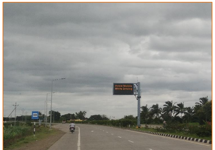
VMS Board at km. 301+100
