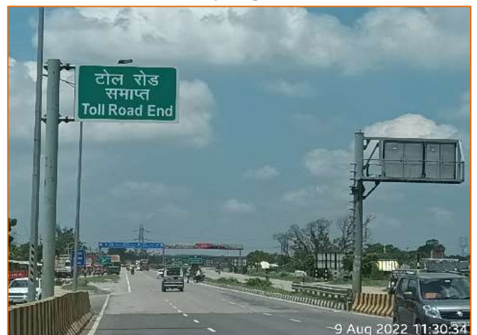
Cantilever Gantry Sign at km. 713+000.
