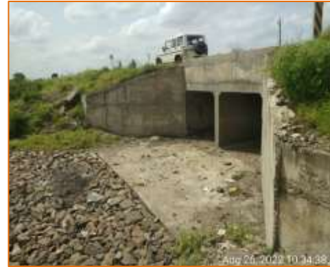
Box culvert at km. 126.643 - RHS (Reconstruction)
