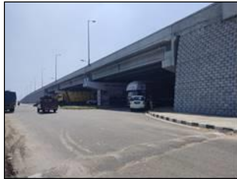
Flyover at km. 39+915
