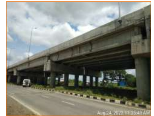
Side View of Flyover at km. 103.801 (LHS)
