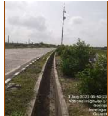
Median longitudinal drain from km. 483+000 to km. 484+000
