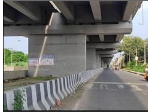
Elevated Structure at km. 25+319
