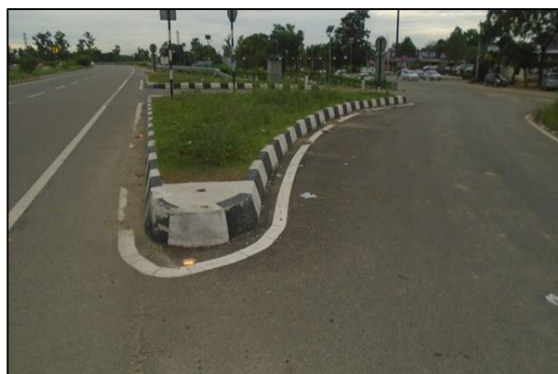
Major Junction at km. 57+260 (RHS)
