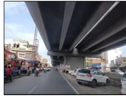
Elevated Structure at km. 25+319
