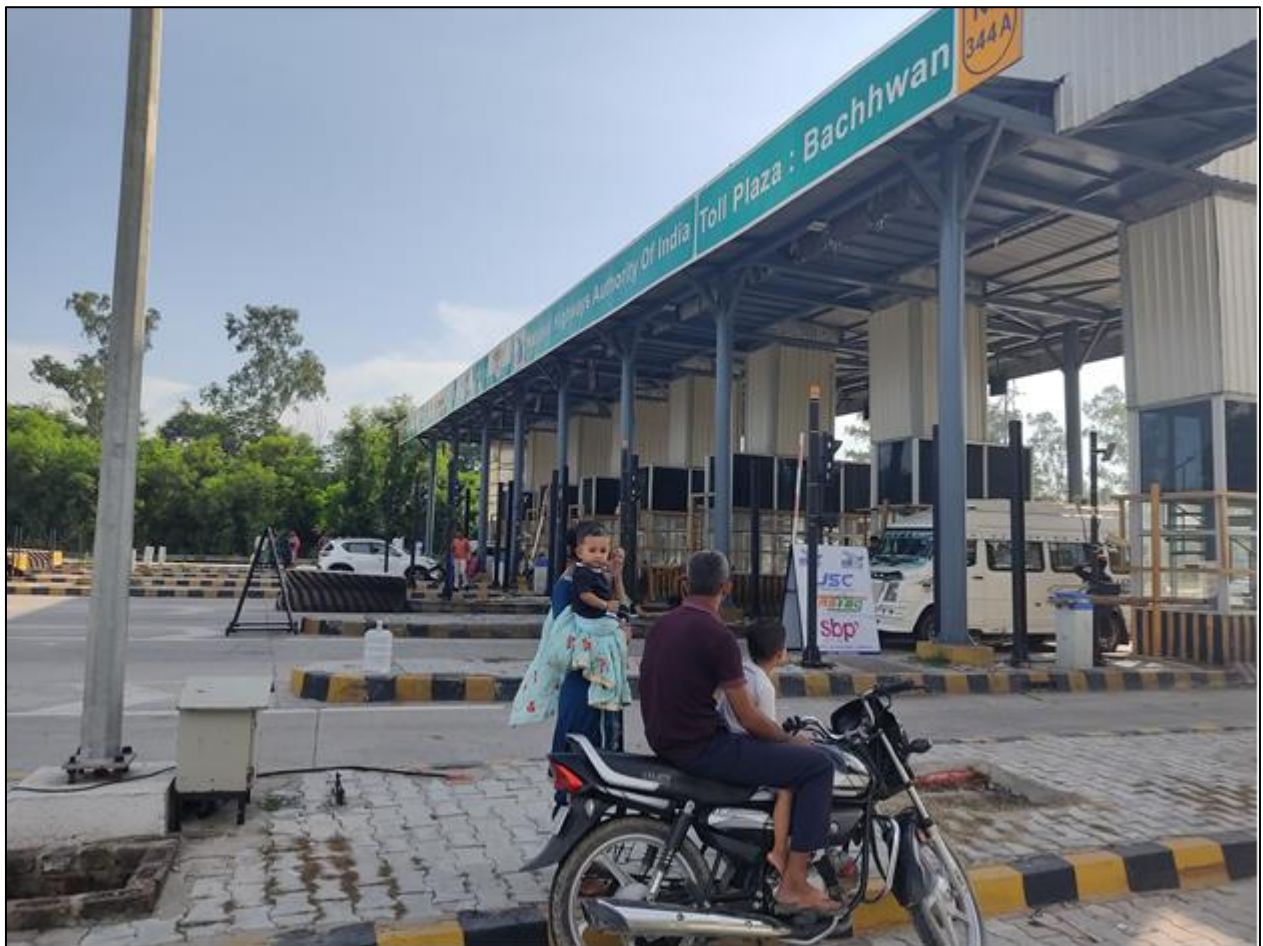
Figure 9-2 View of Bachhwan Toll Plaza (km. 70+240)
