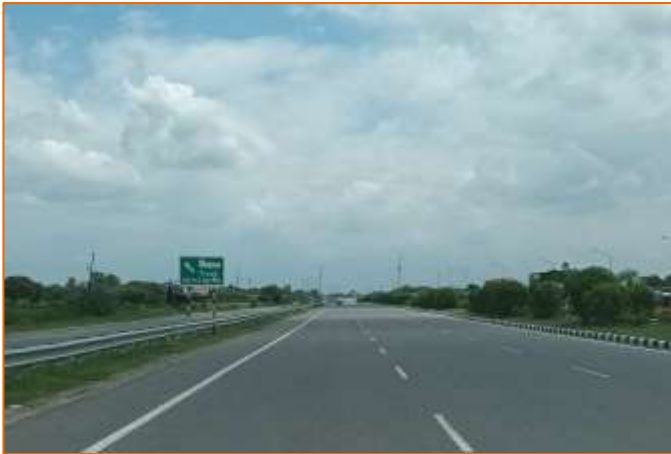
Truck Lay Bye at km. 727+900
