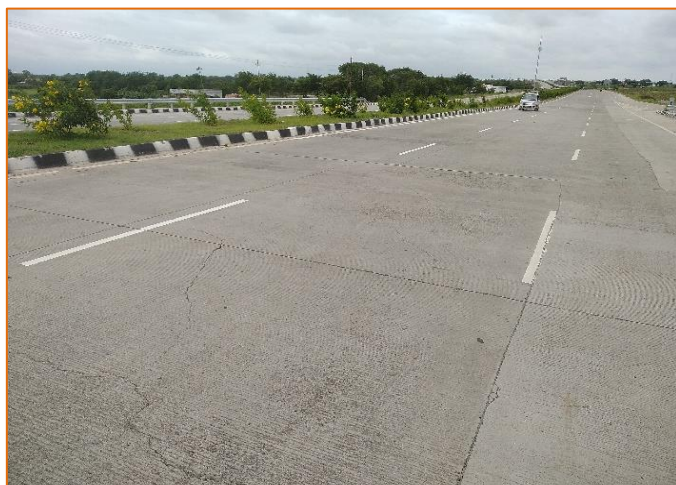
Road Markings at km. 306+500
