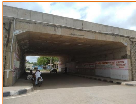
Light Vehicular Underpass at km. 278.700
