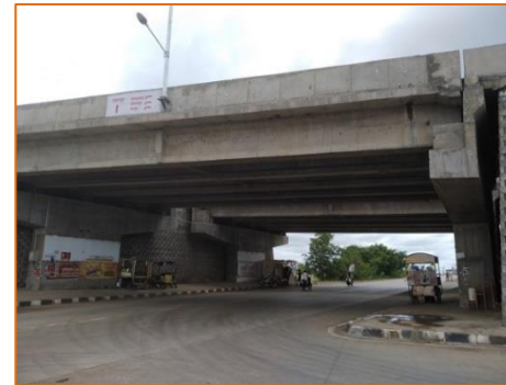
Vehicular Underpass at km. 294.456
