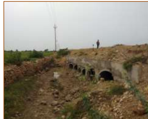
HPC at km. 456+200 (LHS)
