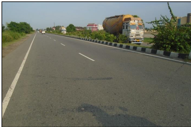
Pavement Condition at km. 6+950
