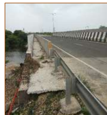
MJB at km. 456+533 (RHS)
