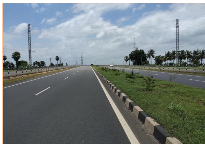
Pavement Condition at km. 76+900
