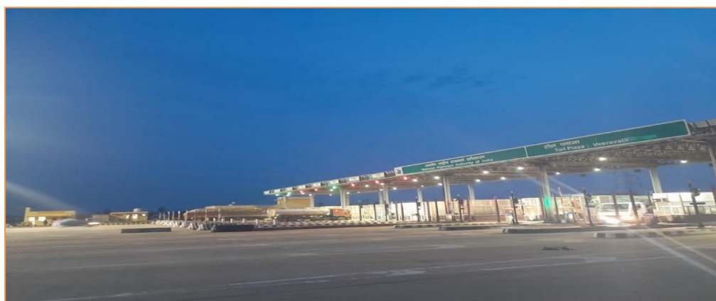
Figure 3-13 View of Toll Plaza
