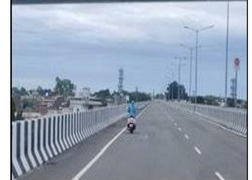
Elevated Structure at km. 25+319
