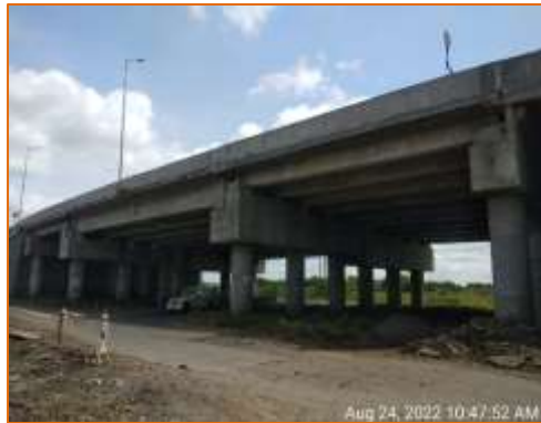
Side View of Flyover at km. 99.900 (LHS)
