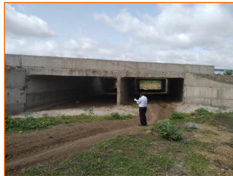
New Minor Bridge at km. 296.580
