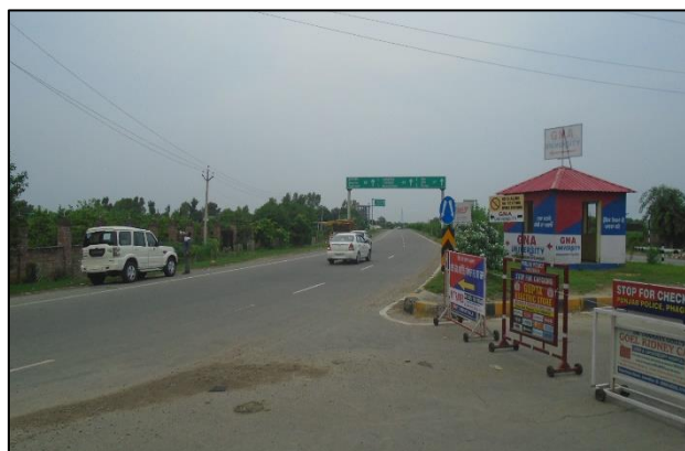
Start of Project Road - Left Carriageway
