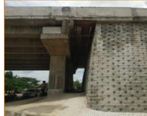
De-shuttering at bottom @ A1 & A2 Side of Flyover at km. 117.935 (RHS)
