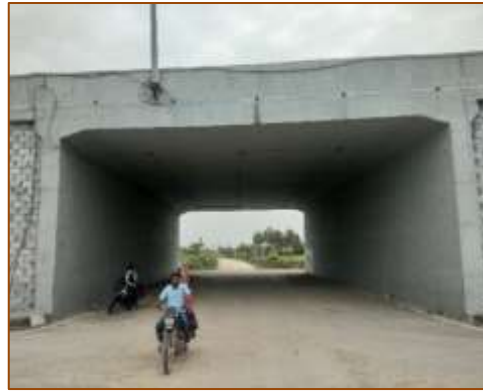
LVUP at km. 381+600 (LHS) - Under COS
