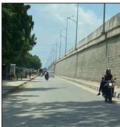
Service Road at km. 765+150
