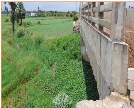
View of Minor Bridge at km. 24+603
