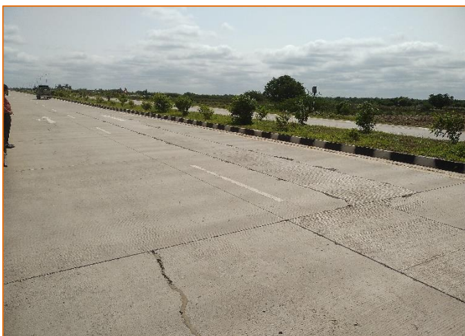
Panel Repair work done at km. 276+050 (LHS)
