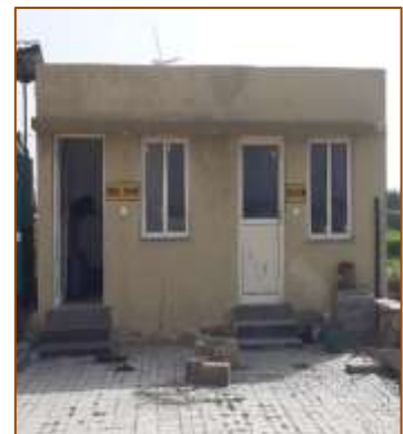
Panel / Pump Room
