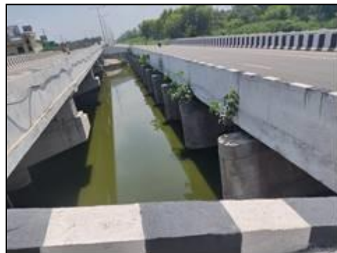
Major Bridge at km. 59+381 (Top View)
