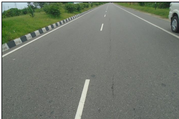
Pavement Condition at km.33+000
