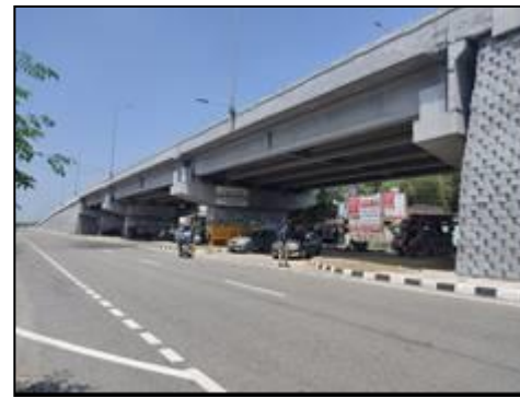
Flyover at km. 59+818
