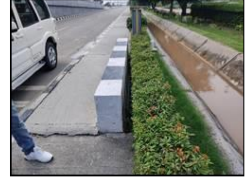
HP Culvert at km. 6+874
