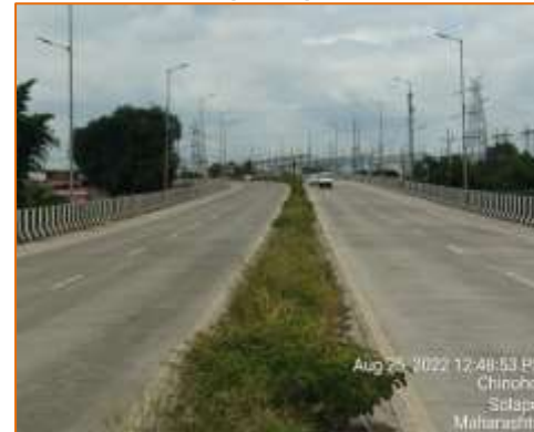
Good condition of PQC surface of MNB at km. 121.678 - BHS (MCW)
