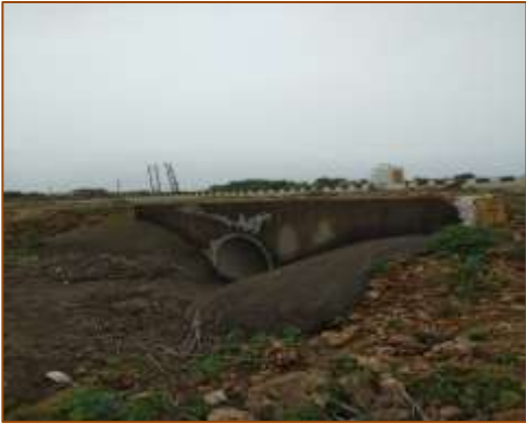
HPC at km. 380+328 (LHS)
