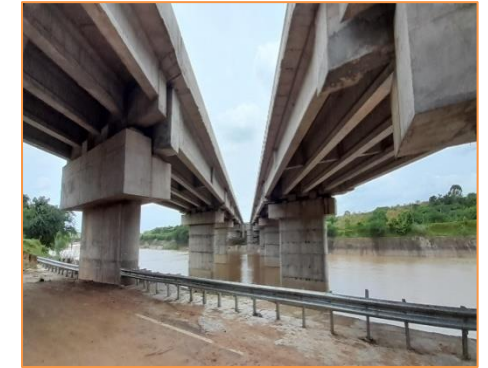
View of Major Bridge at km. 68+742
