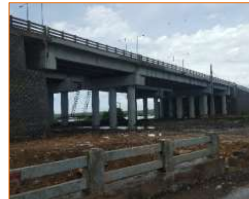
Side View of ROB at km. 0+527 (RHS)
