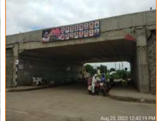
Side View of LVUP at km. 121.950 (LHS)
