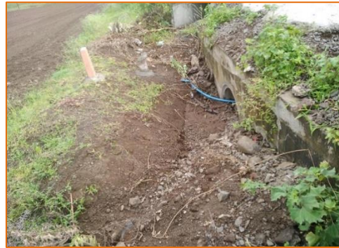
Pipe Culvert at km. 299+507
