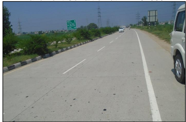
Rigid Pavement at km. 41+000
