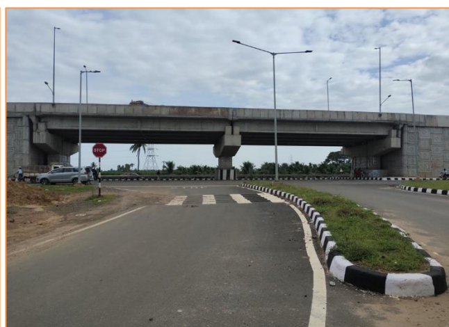
End of Project Road km. 48+830
