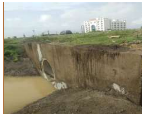
HPC at km. 490+350 (LHS)
