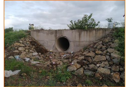
Pipe culvert at km. 310+423
