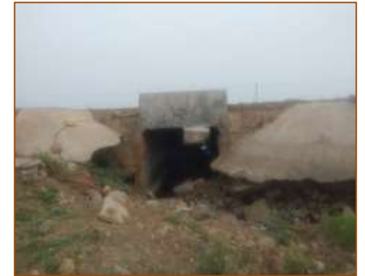
Slab culvert at km. 441+648 (RHS)
