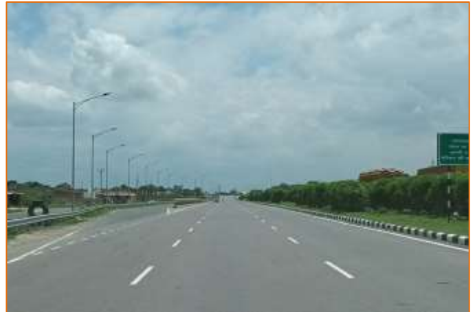
Truck Lay Bye at km. 767+330
