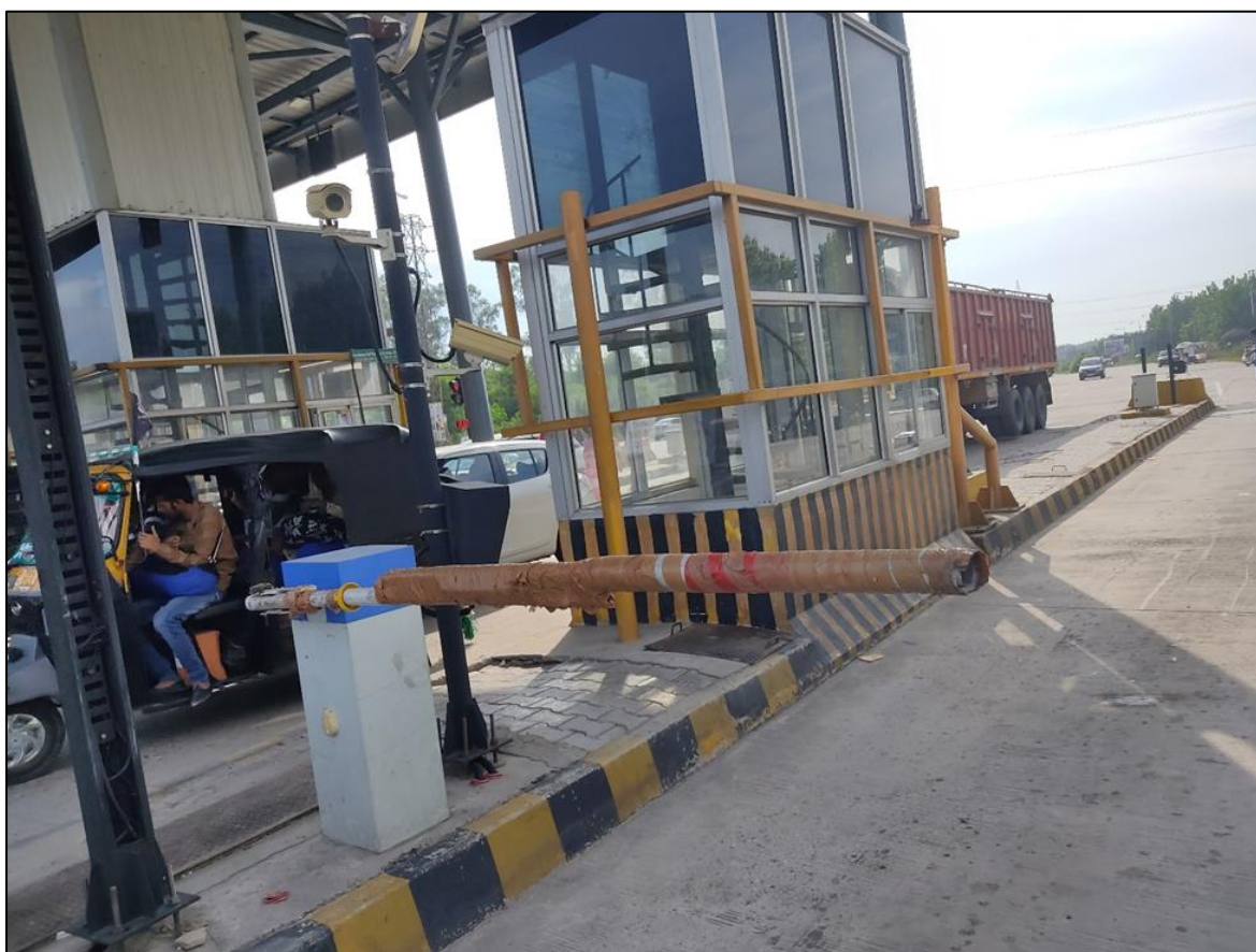
Figure 9-7 Automatic Lane Barrier
