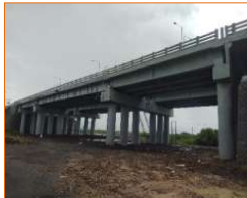
Side View of ROB at km. 0+527 (LHS)
