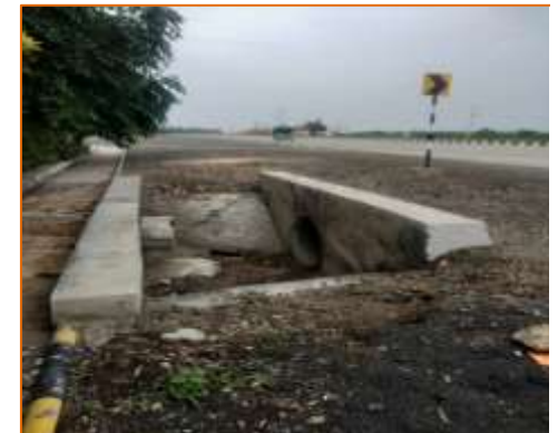
HPC at km. 70+640 (LHS)
