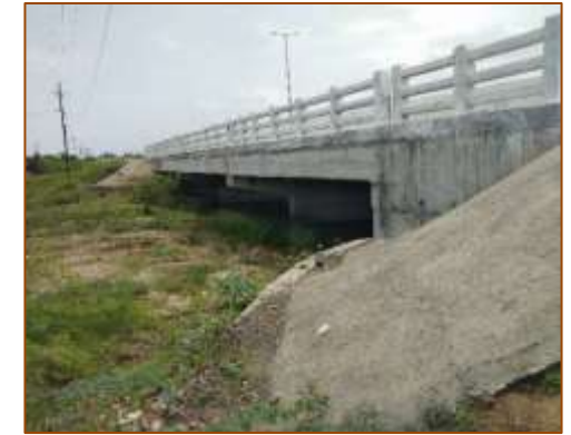
Side view of Minor Bridge at km. 434+974 (LHS) - Widening
