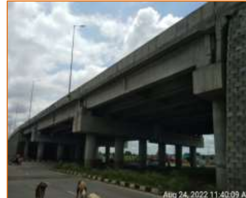
Side View of Flyover at km. 103.801 (RHS)
