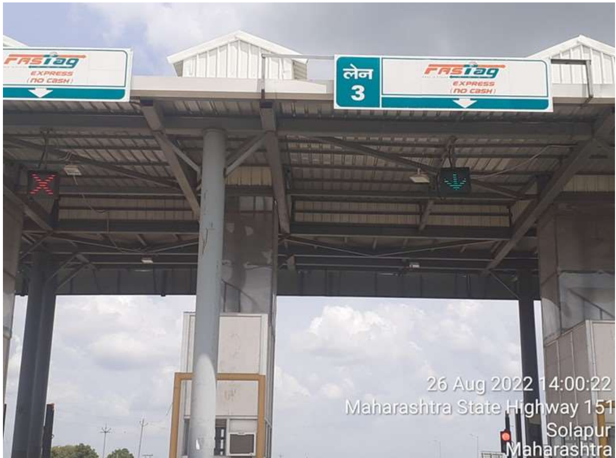
Figure 9-5 OHLS indicating green arrows for operational lanes
