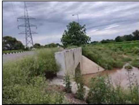
Box Culvert at km. 17+946
