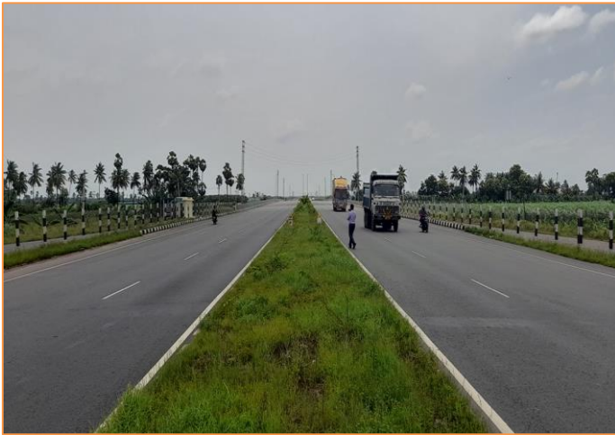
Pavement Condition at km. 41+200
