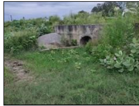
HP Culvert at km. 1+850
