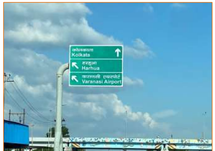
Cantilever Gantry Sign at km. 782+500
