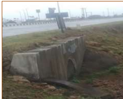
HPC at km. 437+025 (RHS)
