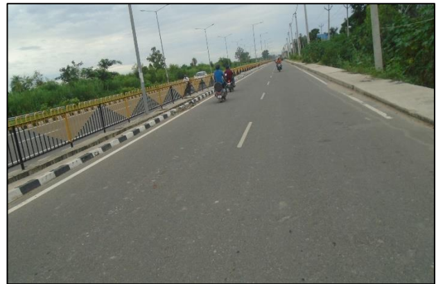
Pedestrian Guard Rail at km. 69+400
