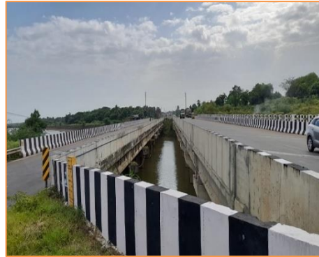
View of Major Bridge at km. 48+222
