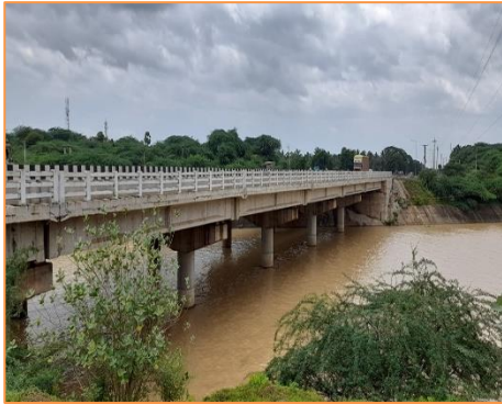
View of Major Bridge at km. 31+647
