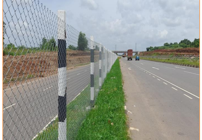
Chain fencing at km. 78+800
