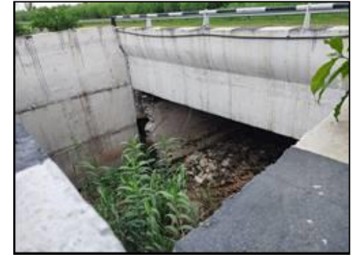
Minor Bridge at km. 76+815 (Structure View)
