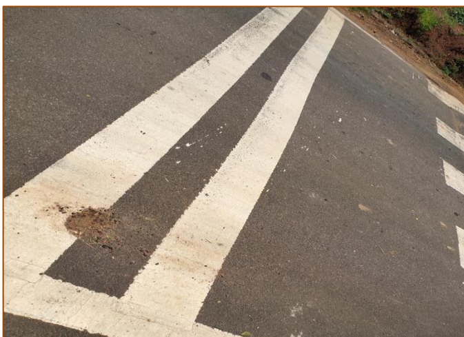
Road Markings at km. 29+400
