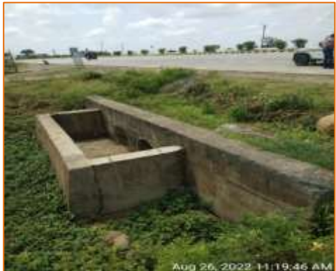
Pipe Culvert at km. 117.423 - RHS (Widening)
