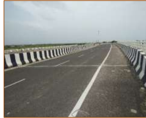
Wearing Coat of MJB at km. 395+255 (LHS)
