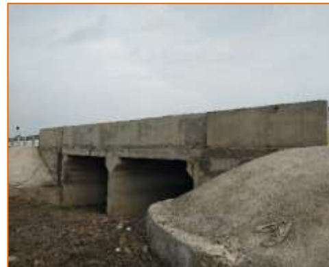
Side View of Minor Bridge at km. 47+700 (LHS)
