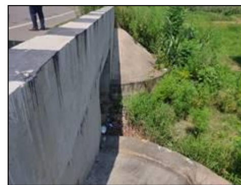
Box Culvert at km. 48+800
