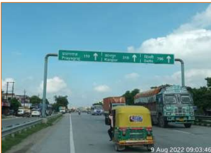
Overhead Gantry Sign at km. 785+040
