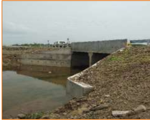
Side View of Minor Bridge at km. 64+765 (LHS)
