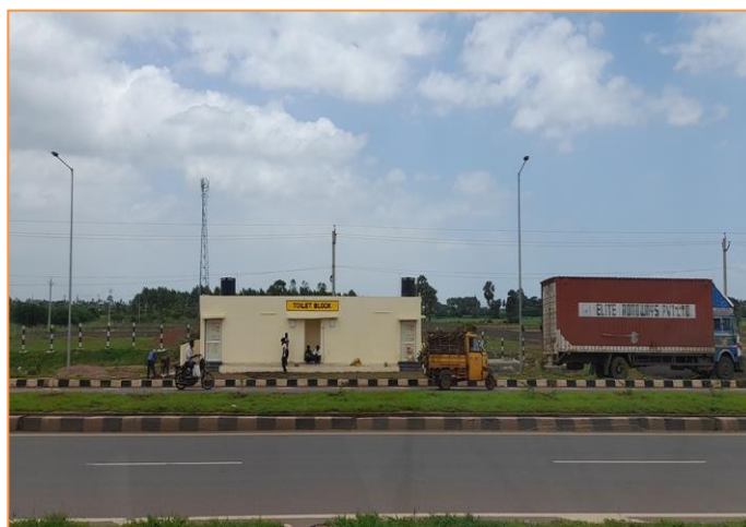
Truck Lay bye at km. 16+520
