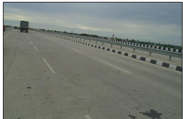
Crash Barrier at curve location
