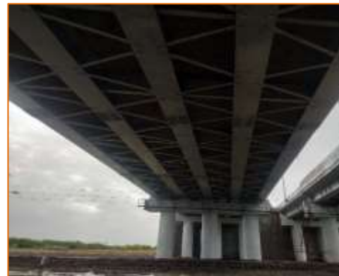
Bottom View of ROB's Girders at km. 0+527
