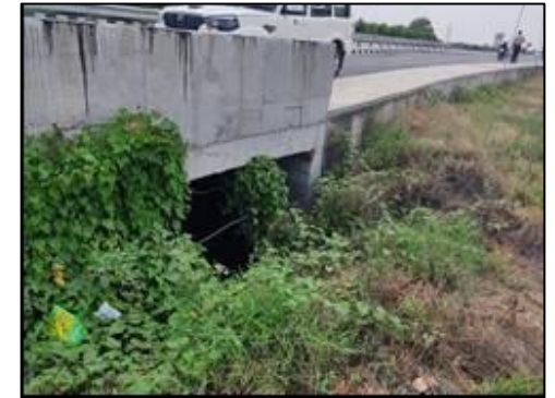
Box Culvert at km. 6+068
