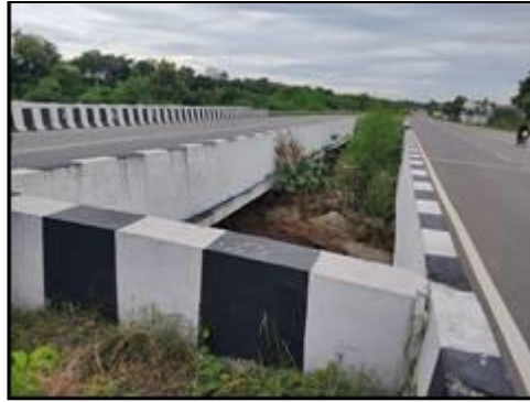
Minor Bridge at km. 72+134 (Top View)
