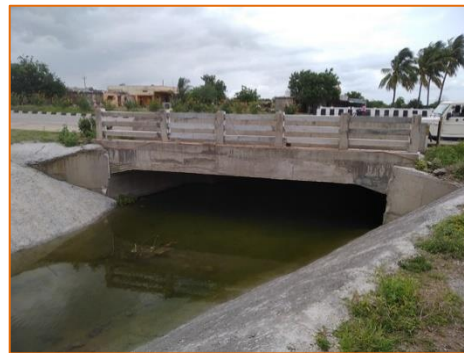
New Minor Bridge at km. 319.849 on LHS
