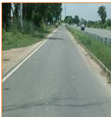
Slip Road at km. 784+400
