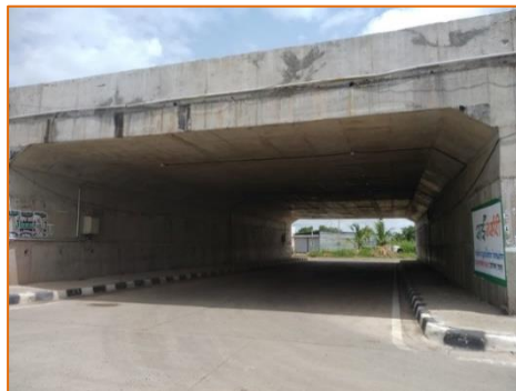
Light Vehicular Underpass at km. 276.900
