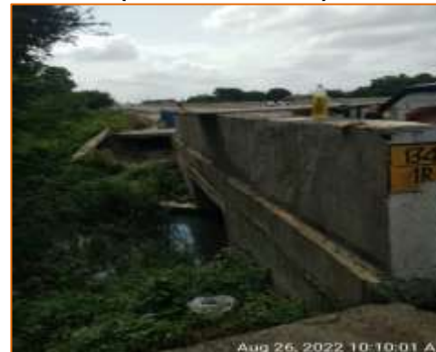
Box culvert at km. 133.524 - RHS (Reconstruction)
