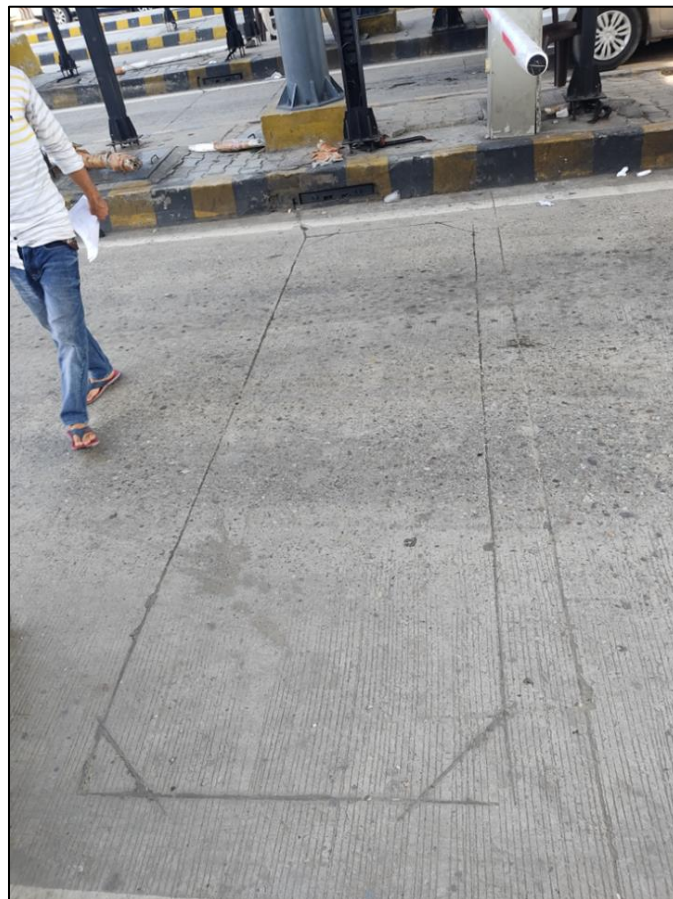
Figure 9-6 Inductive loop
