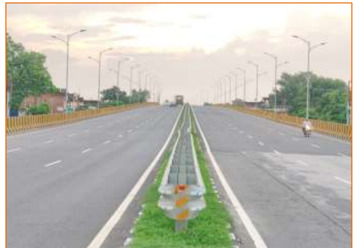
Highway Lighting at km. 740+300
