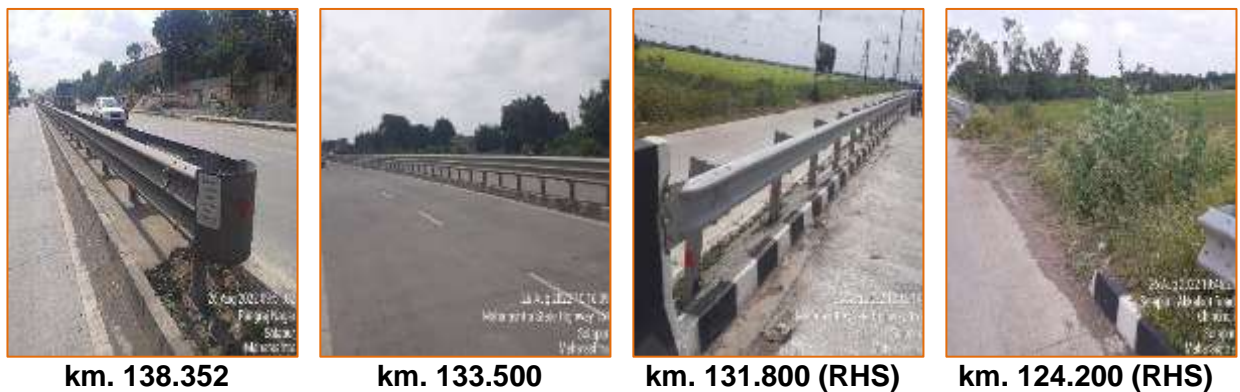
Figure 3-12 Photographs of Crash Barriers
