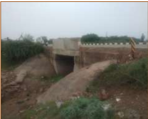
Slab culvert at km. 444+062 (LHS)
