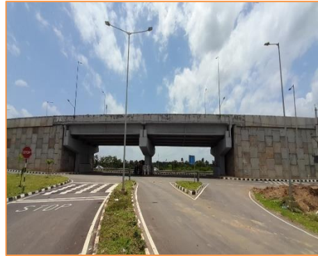
View of UDFO at km. 20+440
