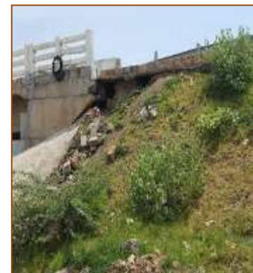
MJB at km. 415+929 (RHS)
