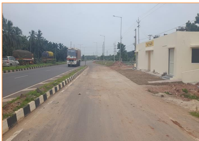
Truck Lay bye at km. 41+500
