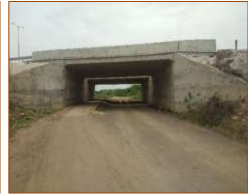
LVUP at km. 488+981 (LHS) - Under COS
