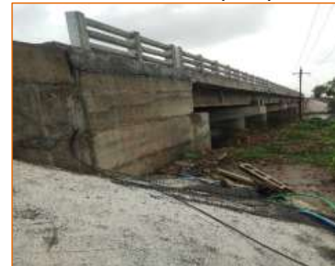
Side View of Major Bridge at km. 23+600 (LHS)
