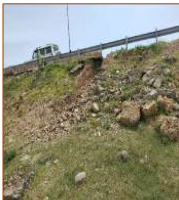
MJB at km. 415+929 (RHS)
