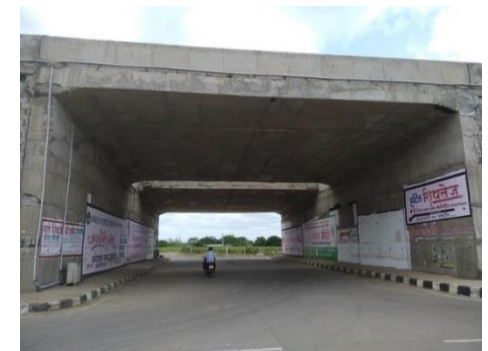
Vehicular Underpass at km. 287.300
