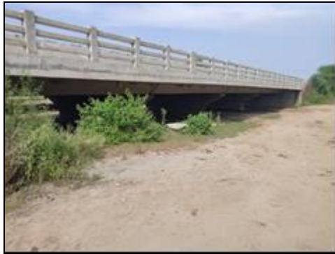
Minor Bridge at km. 68+519 (Existing Structure View)
