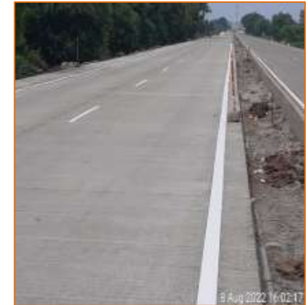
km. 32+450 Work in Progress
