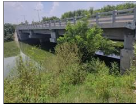
Minor Bridge at km 59+237 (New Structure View)
