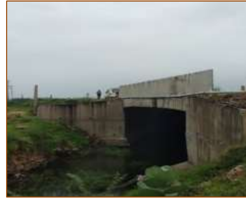
Minor Bridge at km. 385+350 (LHS) - Under COS
