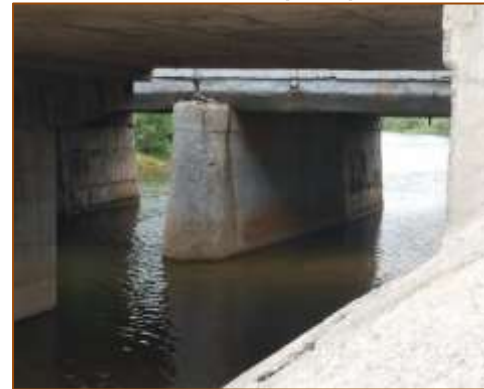
Bottom of Minor Bridge at km. 455+195 (BHS)
