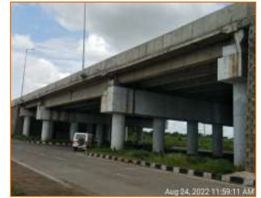
Side View of Flyover at km. 106.240 (LHS)
