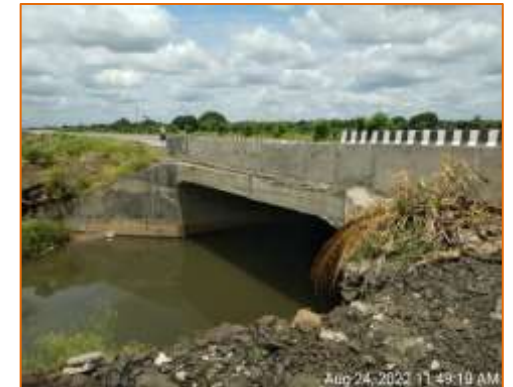
Side View of Minor Bridge at km. 104.348 (LHS)
