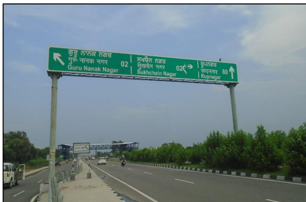
Overhead Gantry Sign Board at km. 8+400
