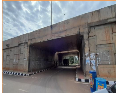
View of LVUP at km 36+420
