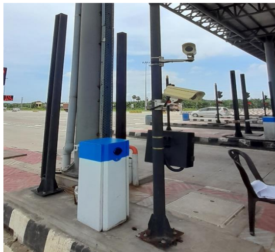
Figure 9-8 LPIC and AVC Cameras
