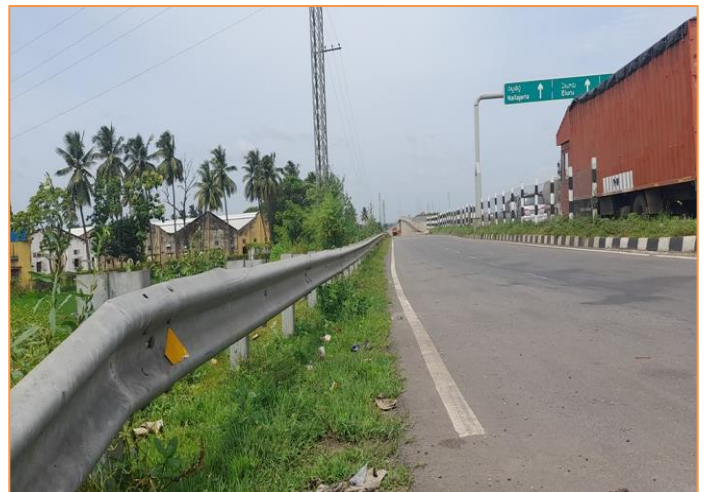
W beam Crash Barrier at km. 85+204
