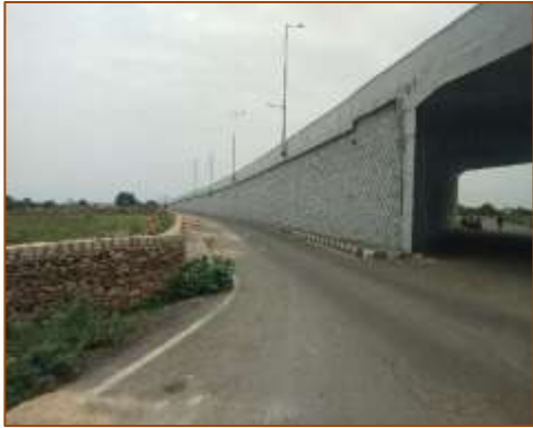
VUP at km. 397+096 (RHS) - Skew - A1 side
