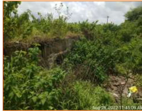
Pipe Culvert at km. 109.578 - LHS (Widening)
