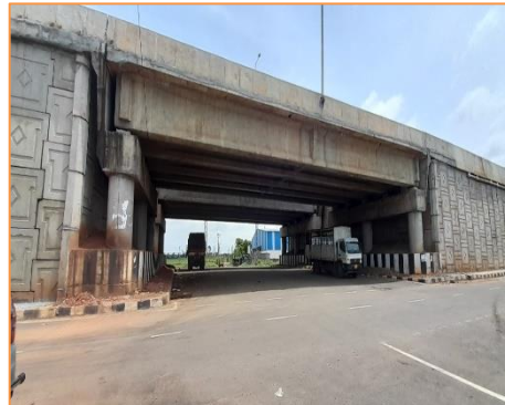
View of VUP at km 83+405
