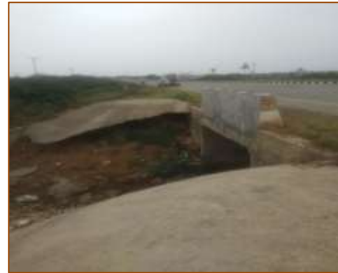
Slab culvert at km. 441+648 (LHS)
