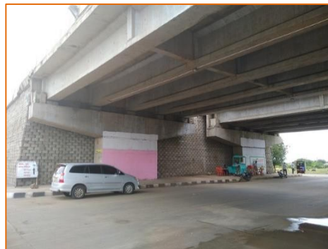
Vehicular Underpass at km. 292.230
