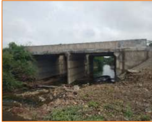
Side View of Minor Bridge at km. 49+243 (RHS)
