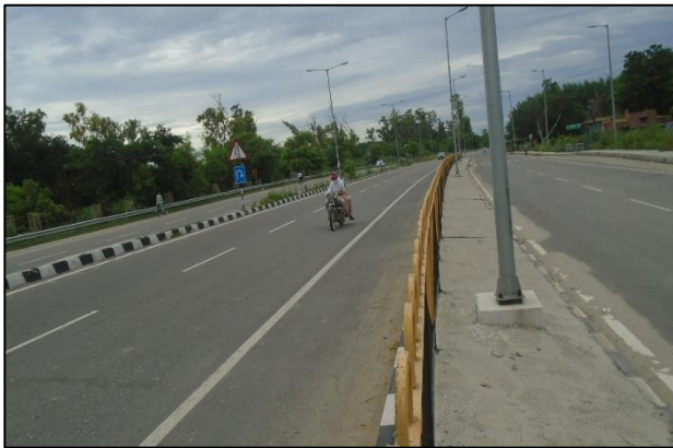
Pedestrian Guard Rail at km. 69+400
