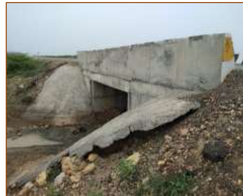
Slab culvert at km. 475+860 (LHS)
