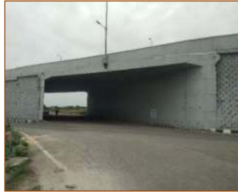
VUP at km. 397+096 (RHS)
