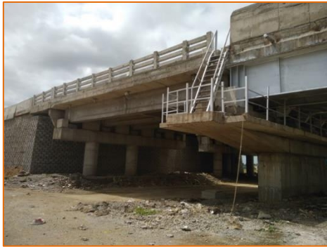
Rail Over Bridge at km. 294.125
