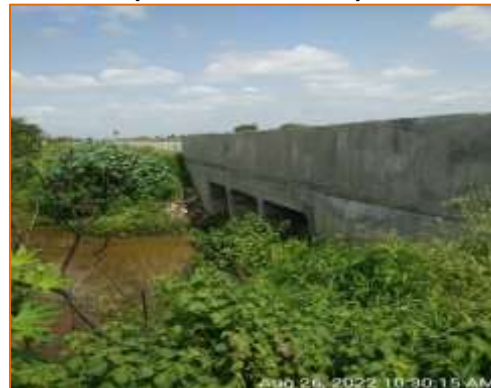
Box culvert at km. 128.229 - LHS (Reconstruction)
