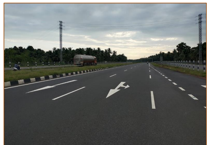
Road Markings at km. 56+760
