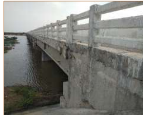
Side View of Major Bridge at km. 389+295 (RHS)
