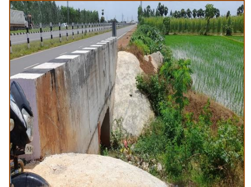
Box Culvert at km. 56+650
