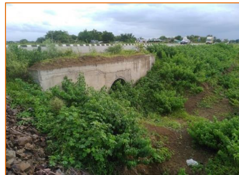
Pipe culvert at km. 318+657
