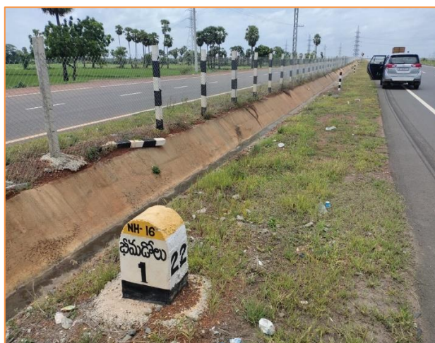
Kilometer stone at km 22+000
