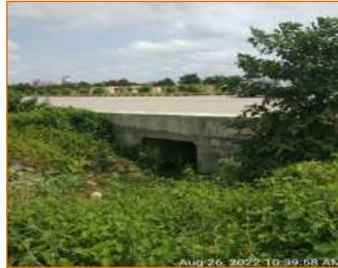
Box culvert at km. 125.495 - LHS (Reconstruction)
