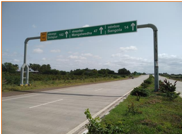
Start of Project Road at km. 276.000
