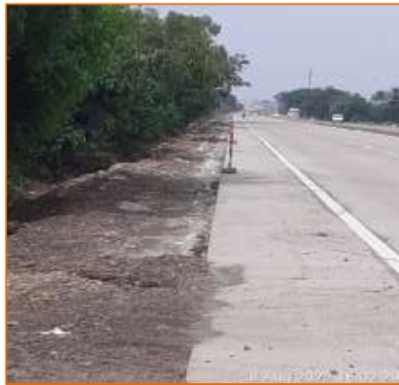
km. 32+450 Work in Progress
