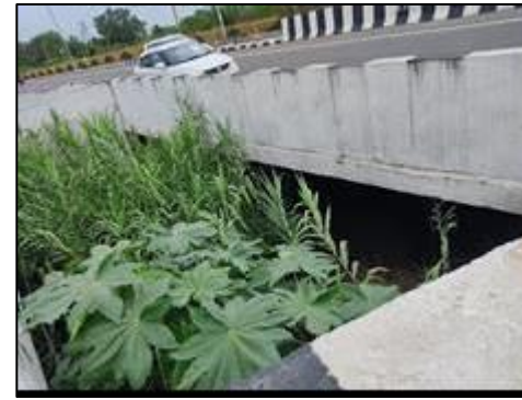
Minor Bridge at km. 78+636 (Structure View)
