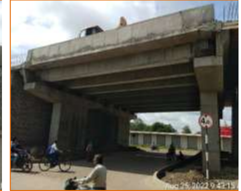
Side View of PUP at km. 136.657 (RHS)
