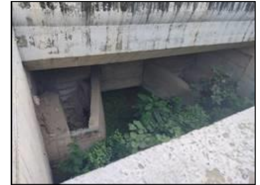
Minor Bridge at km. 69+815 (Existing Structure View)
