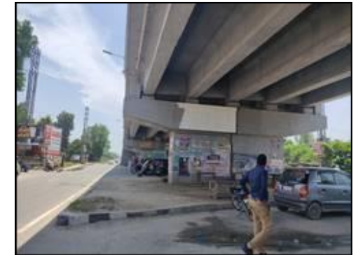
Flyover at km. 59+818
