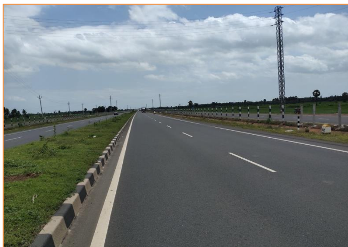
Pavement Condition at km. 71+300
