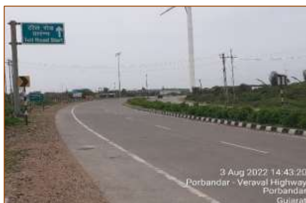
Porbandar Bypass at km. 379.100
