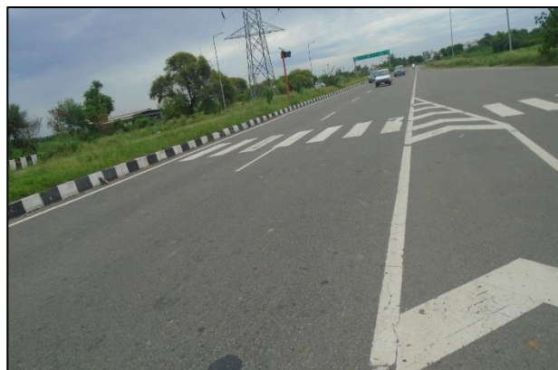
Road Marking at km. 15+800 (RHS)
