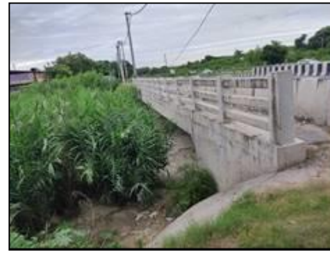
Minor Bridge at km. 75+009 (Structure View)
