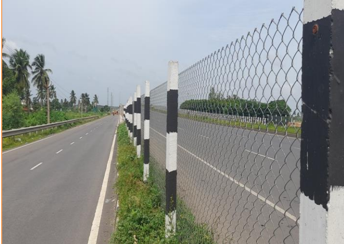
Chain fencing at km. 85+150
