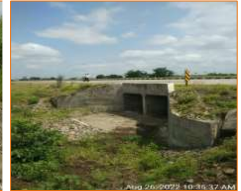
Box culvert at km. 126.643 - LHS (Reconstruction)
