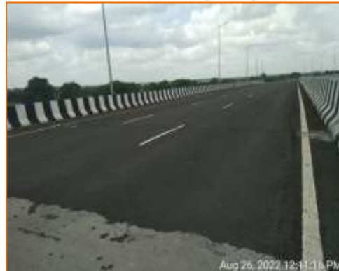
BC surface of Flyover at km. 102.700 (LHS)
