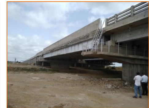
Rail Over Bridge at km. 294.125
