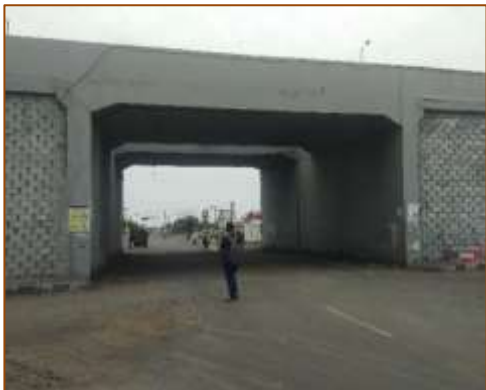
VUP at km. 400+681 (RHS)
