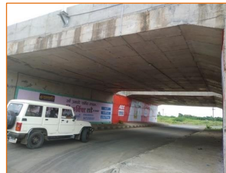
Light Vehicular Underpass at km. 320.900
