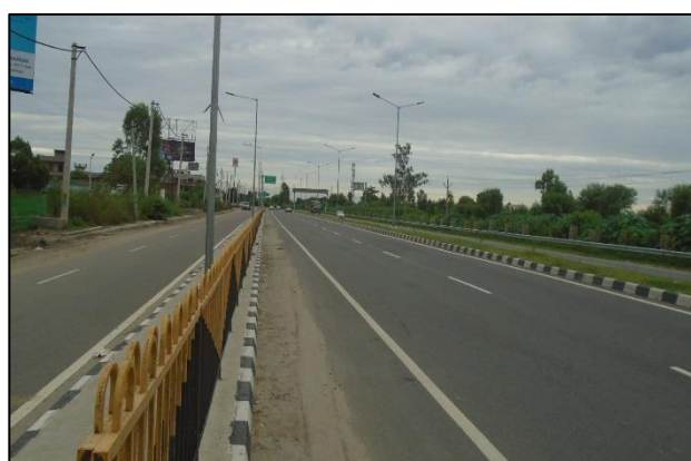
Approach to End of Project Road
