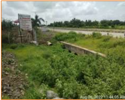
Pipe Culvert at km. 109.578 - RHS (Widening)
