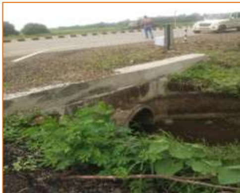
HPC at km. 66+010 (RHS)
