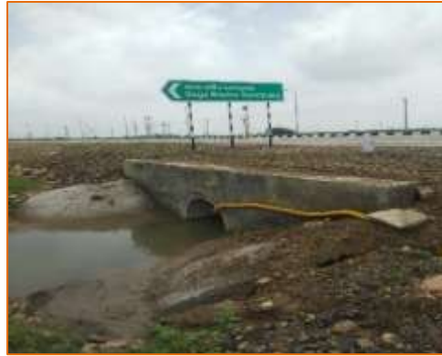
HPC at km. 5+800 (LHS)
