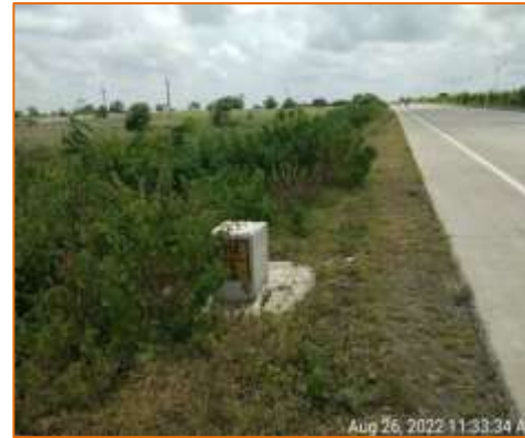
Pipe Culvert at km. 113.155 - RHS (Widening)
