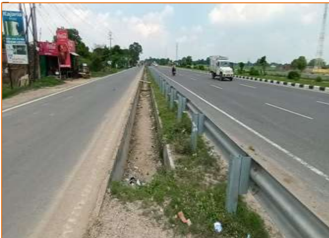
RCC Open Drain at km. 762+000
