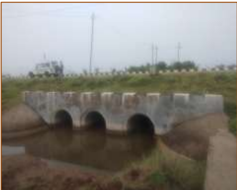
HPC at km. 437+025 (LHS)
