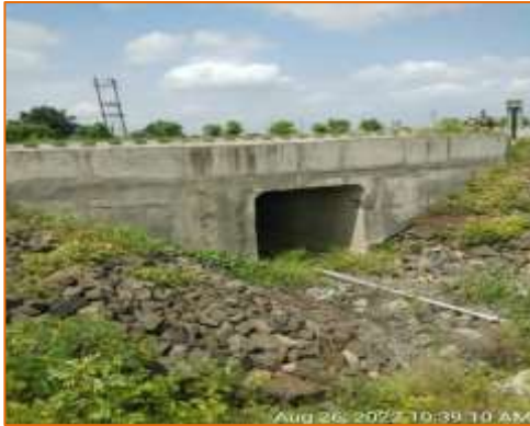
Box culvert at km. 125.495 - RHS (Reconstruction)
