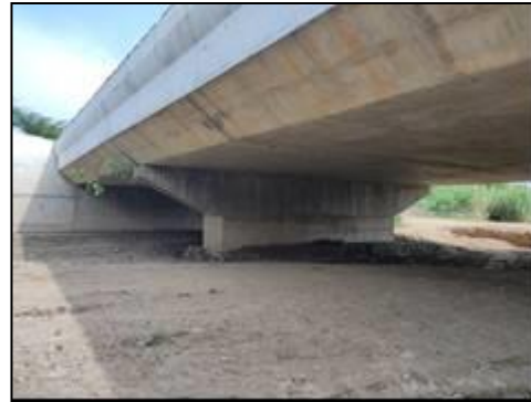
Minor Bridge at km. 68+519 (Substructure and Superstructure)
