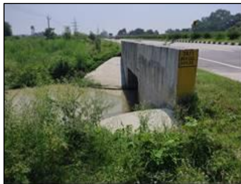
Box Culvert at km. 37+480
