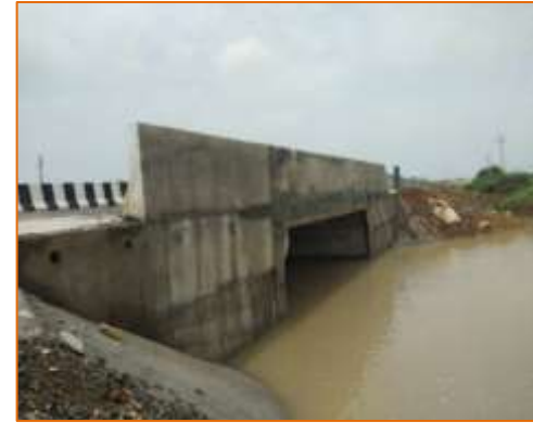
Side View of Minor Bridge at km. 9+880 (LHS)
