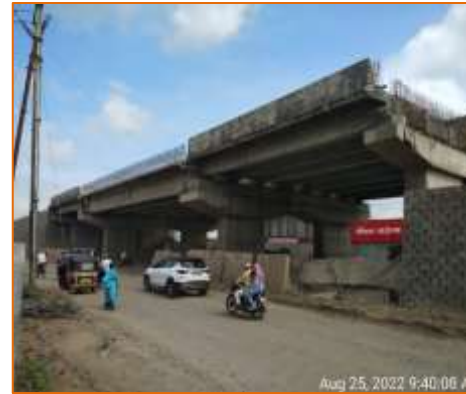
Side View of Flyover at km. 136.857 (LHS)
