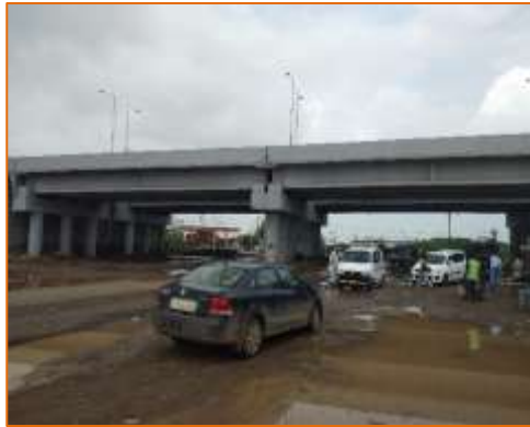
Side View of VUP at km. 12+420 (RHS)
