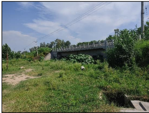
Minor Bridge at km. 62+704 (Existing Structure View)
