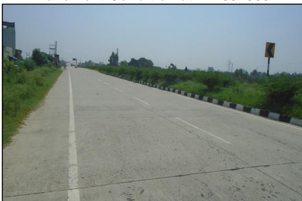
Rigid Pavement at km. 38+000
