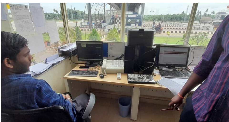
Figure 9-14 Work Stations at Control room
