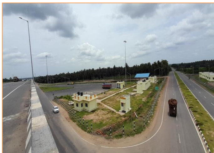
Rest Area at km. 66+800
