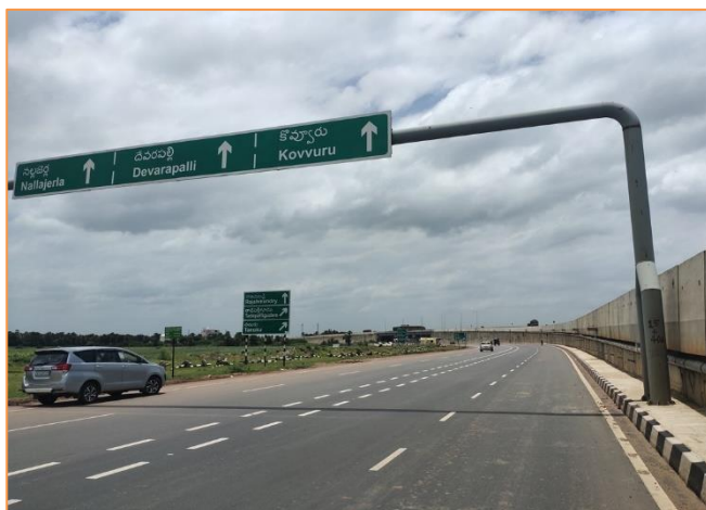
Start of Project Road at km. 15+700
