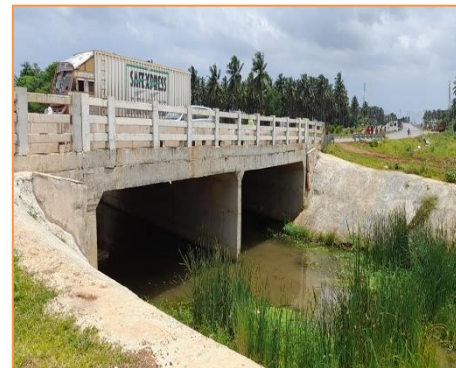
View of Minor Bridge at km. 28+782
