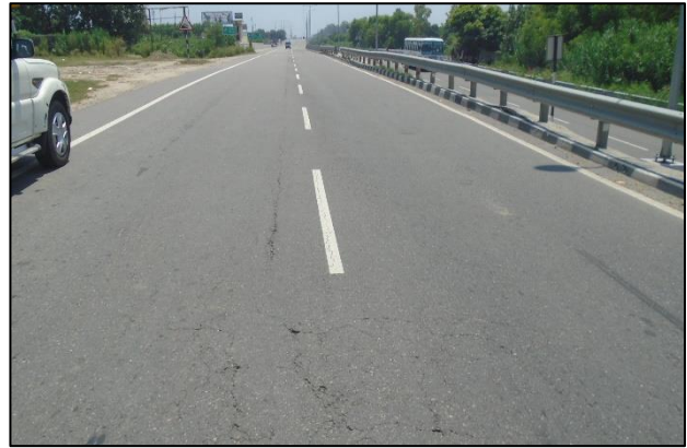
Pavement Condition at km. 59+000
