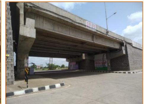
Vehicular Underpass at km. 290.700
