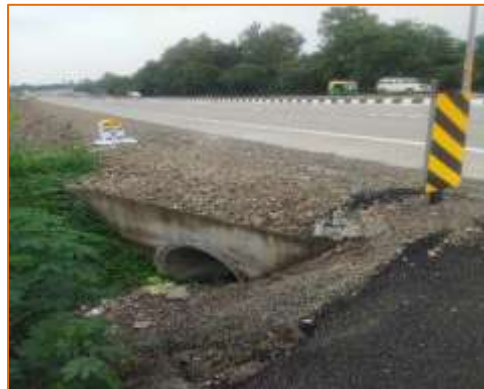
HPC at km. 66+010 (LHS)
