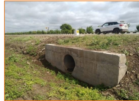
Pipe Culvert at km. 292+135
