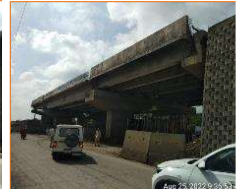
Side View of Flyover at km. 136.857 (RHS)
