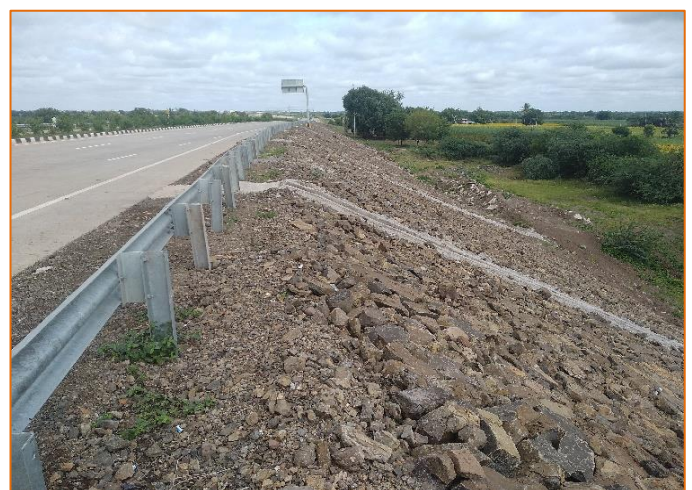
Slope Protection work at km. 298+300
