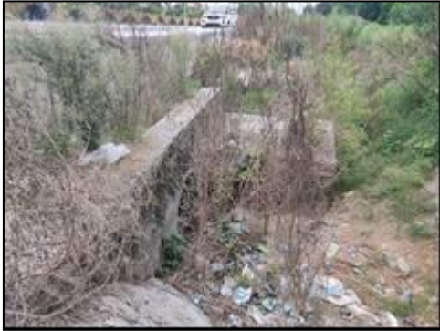
HP Culvert at km. 80+569
