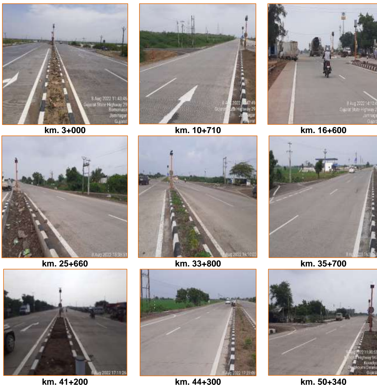
Figure 3-2 Photographs of Minor Intersection
