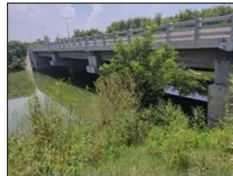
Major Bridge at km. 59+381 (New Structure View)
