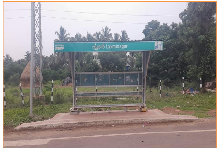
Bus Bay with Shelter at km. 56+140
