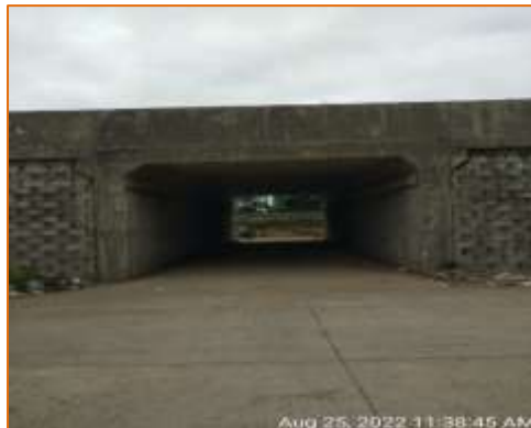
Side View of PUP at km. 130.485 - RHS (Under COS)
