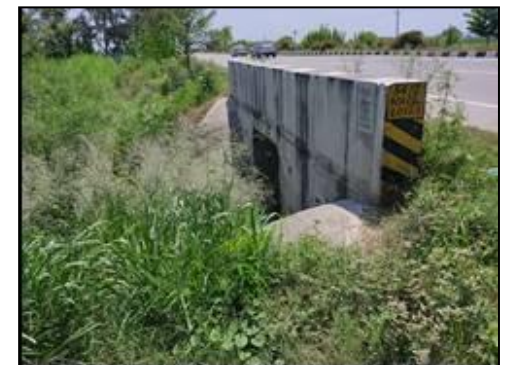
Box Culvert at km. 53+510
