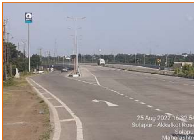
End of the Bypass at km. 106.526
