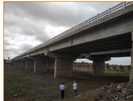
New Major Bridge at km. 298.190
