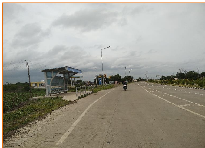
Bus Bay at km. 312+150 (Andhalgaon)
