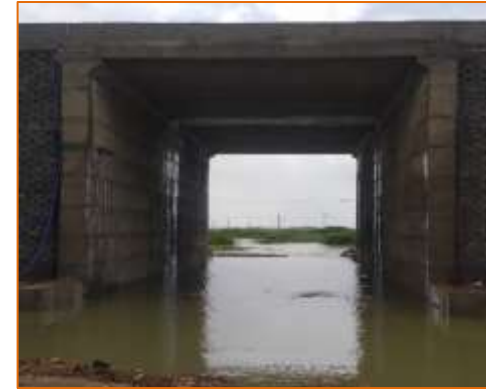
Side View of Minor Bridge at km. 0+580 (LHS)
