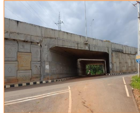
View of LVUP at km 44+135
