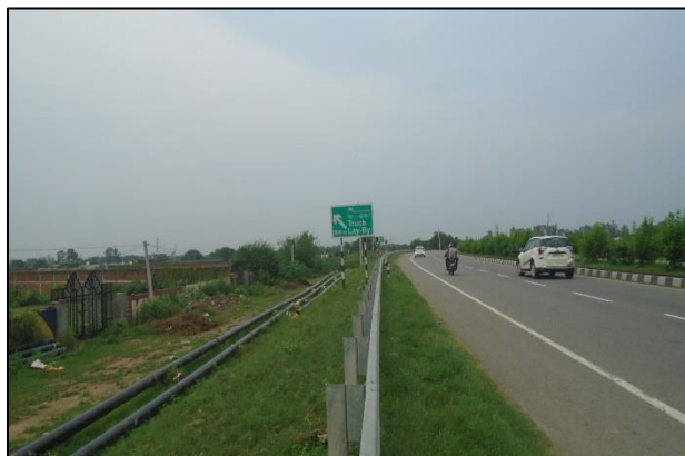
Crash Barrier at high embankment
