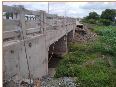
Reconstruction of Minor Bridge at km. 284.835
