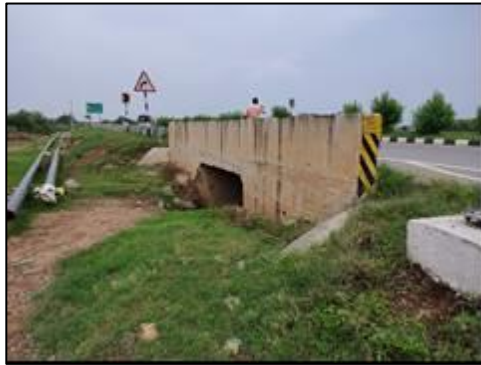
Box Culvert at km. 0+960
