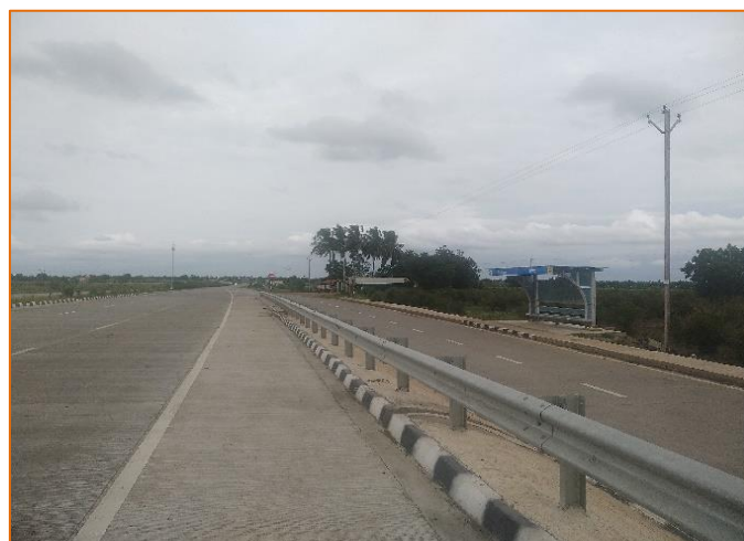
End point of Sangola Bypass at km. 299+150
