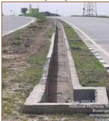
Median longitudinal drain from km. 472+000 to km. 473+000
