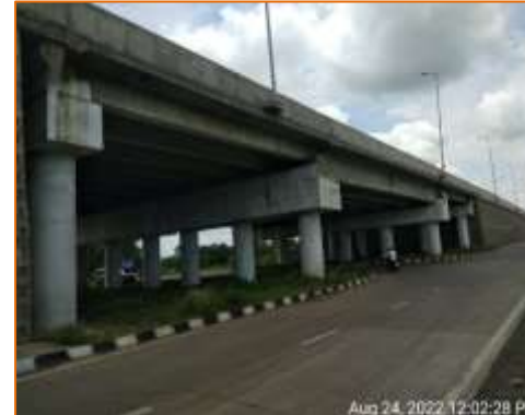
Side View of Flyover at km. 106.240 (RHS)
