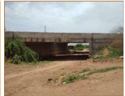
LVUP at km. 488+981 (RHS) - Under COS
