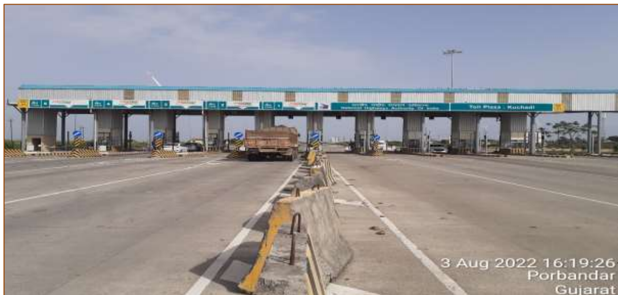
Figure 9-1 View of Kuchadi Toll Plaza (km. 409+500)
