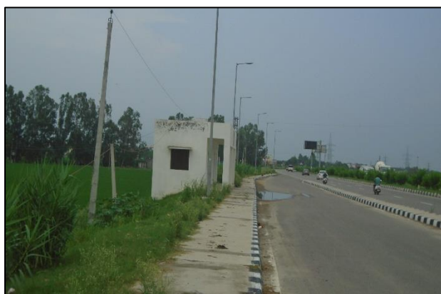
Truck Lay-Bye at km. 1+600
