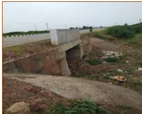
Slab culvert at km. 444+062 (RHS)
