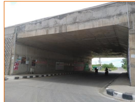
Light Vehicular Underpass at km. 285.432
