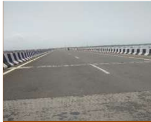
Major Bridge - km. 433+295 (LHS) Wearing Coat
