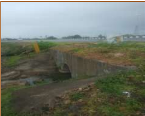
HPC at km. 437+025 (LHS)
