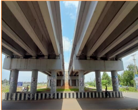
View of Flyover at km. 23+164
