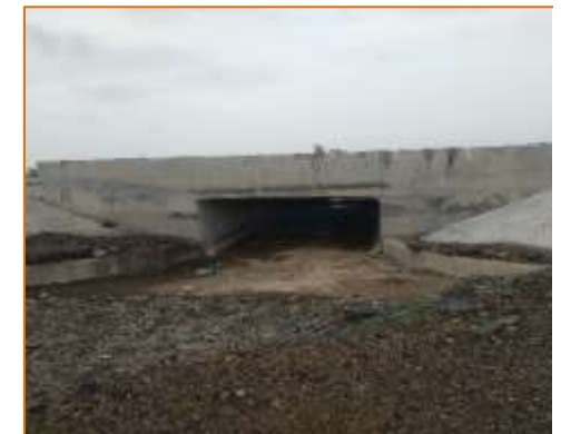
Box culvert at km. 62+720 (RHS)
