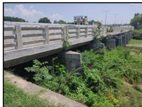
Major Bridge at km. 59+381 (Existing Structure View)
