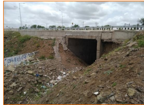
Box Culvert at km. 284+112
