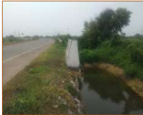
Slab culvert at km. 439+458 (RHS)
