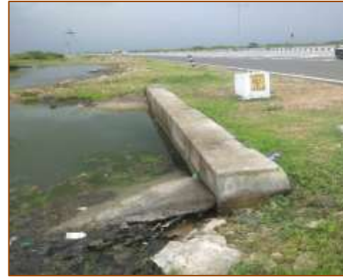
HPC at km. 391+096 (LHS)
